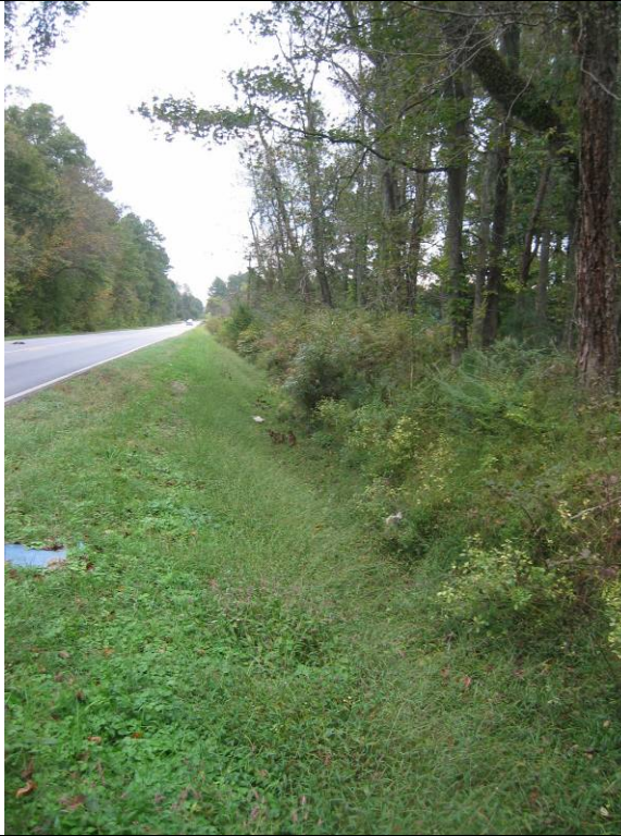
Photo 7: Road side ditch flowing to north section of TOM-A tract (10/18/04 – Typical)
