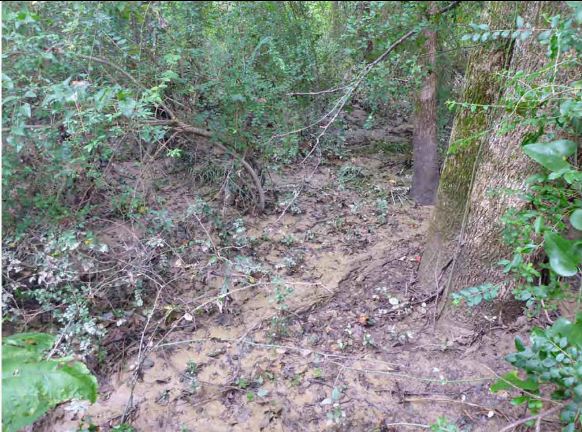
WP7 (September 10, 2014) Northern breach in berm from Swift Creek
