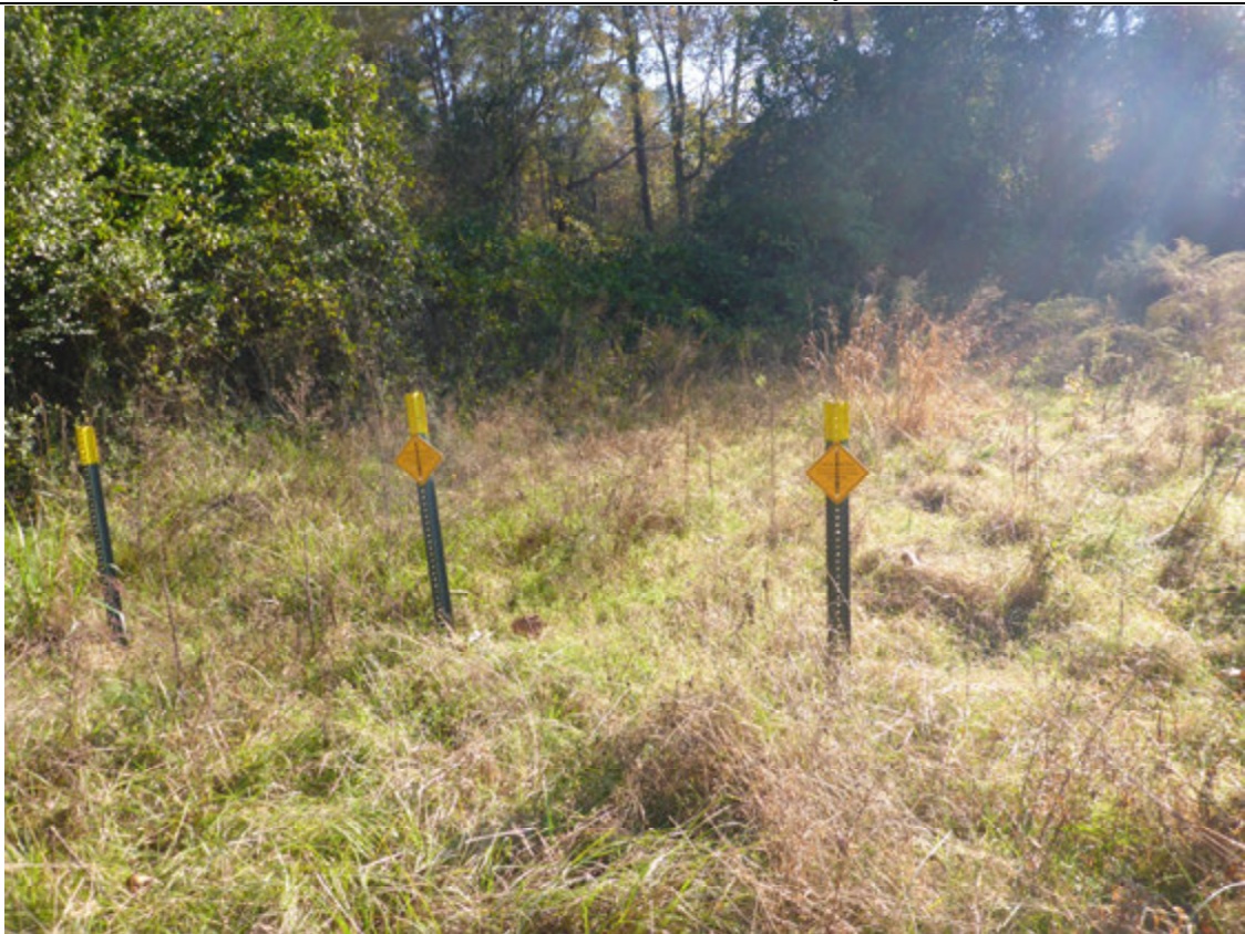
WP6 (November 12, 2015) Secondary barrier constructed in easement encroachment
