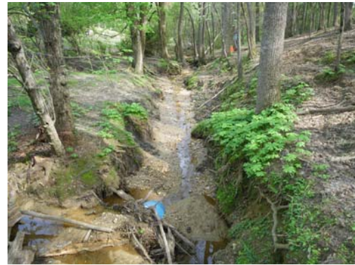
Cow Tributary 2, looking downstream; bank erosion and channel incision; February 8, 2011
