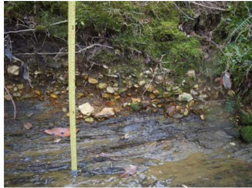
Moores Fork, near station 60+00; bank erosion; channel incision; January 16, 2012
