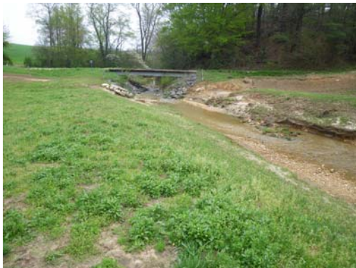
Moores Fork, looking downstream from station 34+00; clear-span bridge, riprap armor; April 20, 2011
