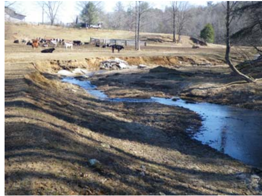
Moores Fork; looking downstream from station 18+50; direct cattle access; bank erosion; February 8, 2011
