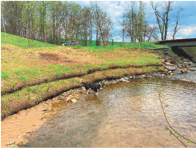
Moore's Fork Reach 2 STA 35+40 left bank repair – 4/19/2021
