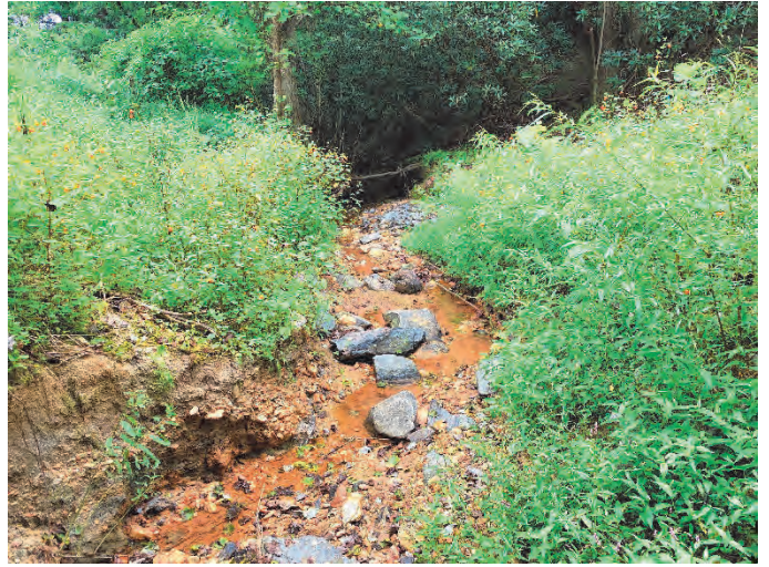
Silage Reach 1 STA 19+00 right bank repair – 9/8/2021
