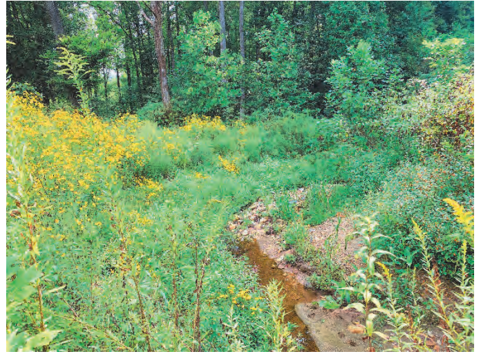
Silage Reach 1 STA 30+30 left bank repair – 9/8/2021
