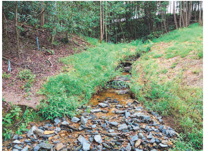
UT1 downstream repair near confluence with Silage Reach 1 – 9/8/2021
