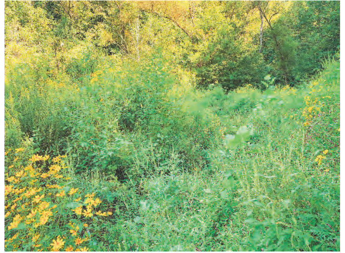
UT10/Wetland outlet repair – 9/7/2021
