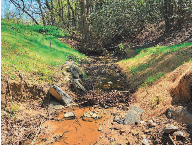
Silage Reach 1 STA 19+00 right bank repair – 4/20/2021
