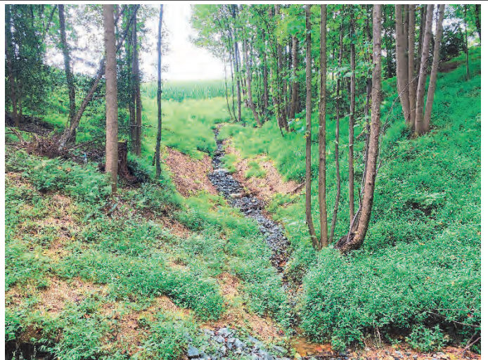
Upper UT1 repair area gully stabilization – 9/8/2021
