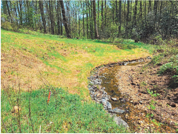
Silage Reach 1 STA 30+30 left bank repair – 4/20/2021
