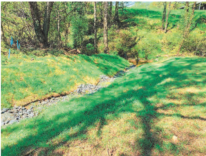
Silage Reach 1 STA 10+40 gully stabilization – 4/19/2021
