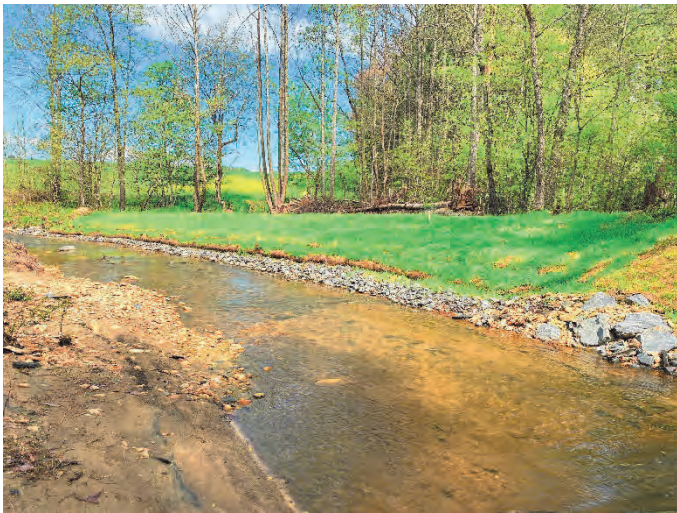
Moore's Fork Reach 3 STA 64+10 left bank repair – 4/19/2021
