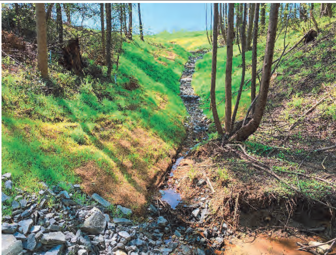
Upper UT1 repair area gully stabilization – 4/20/2021
