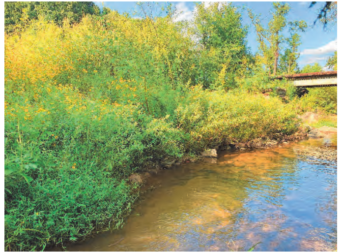
Moore's Fork Reach 2 STA 35+40 left bank repair – 9/7/2021
