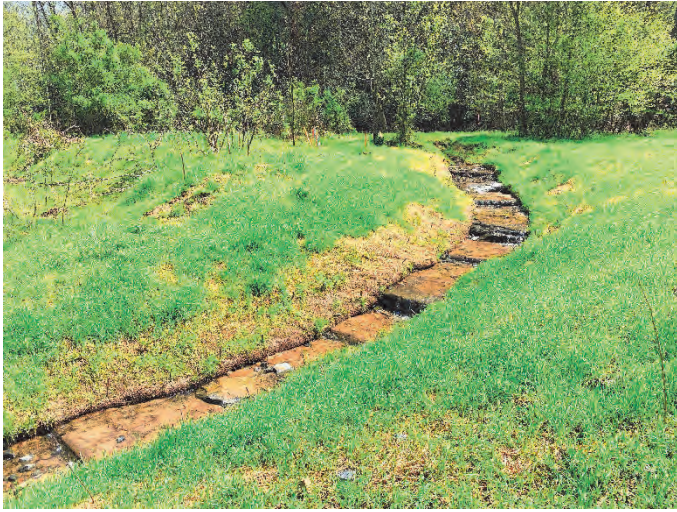
UT10/Wetland outlet repair – 4/19/2021
