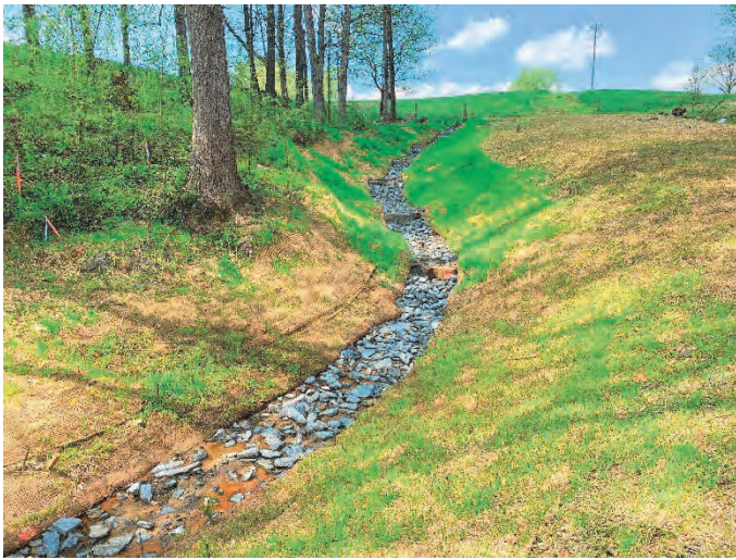
Upper Cow Trib 2 repair area gully stabilization – 4/20/2021
