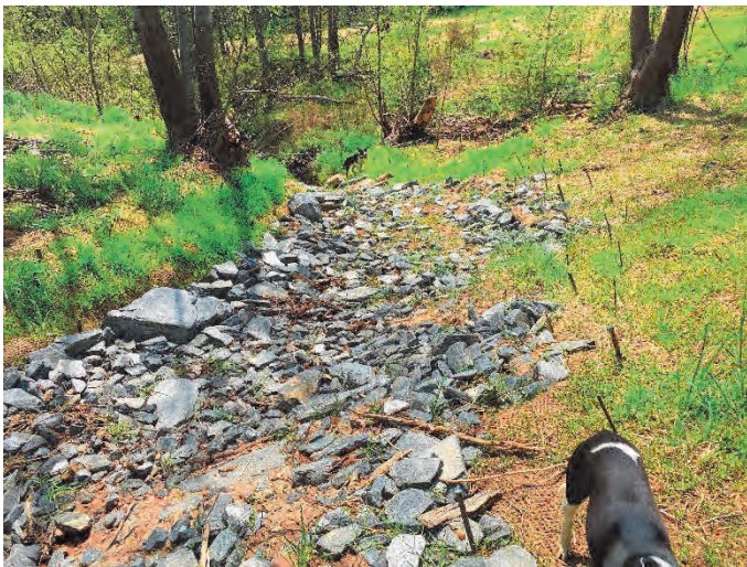
Upper Cow Trib 2 repair area – 4/20/2021
