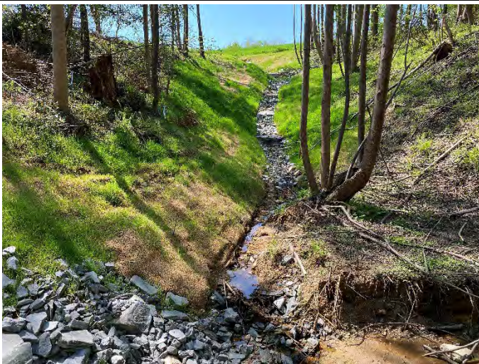
Upper UT1 repair area gully stabilization – 4/20/2021
