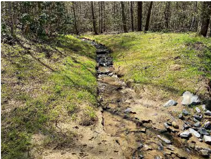
UT8/Wetland outlet repair at confluence with Moore's Fork – 4/19/2021
