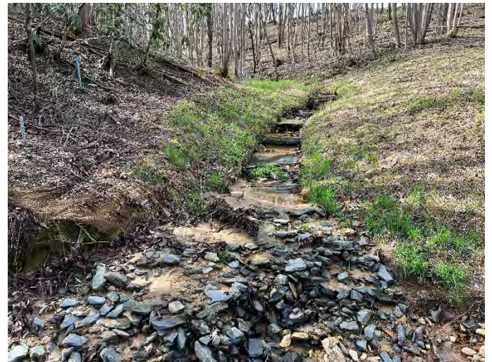
UT1 downstream repair near confluence with Silage Reach 1 – 4/06/2022
