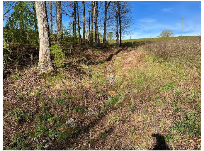
Upper Cow Trib 2 repair area gully stabilization – 4/06/2022
