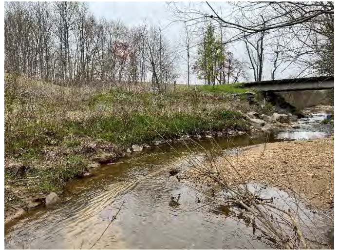
Moore's Fork Reach 2 STA 35+40 left bank repair – 4/05/2022
