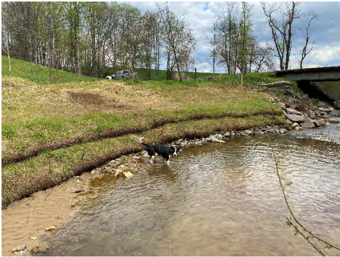
Moore's Fork Reach 2 STA 35+40 left bank repair – 4/19/2021
