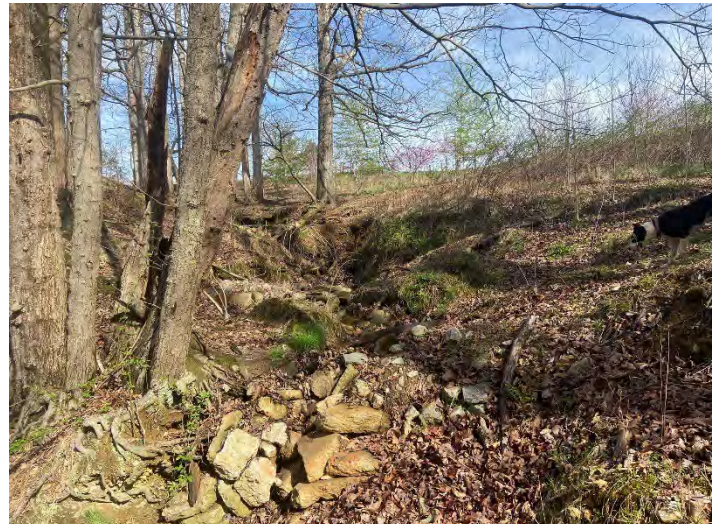
PP50 – Cow Tributary 1, looking upstream (04/06/2022)
