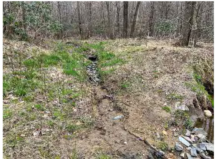
UT8/Wetland outlet repair at confluence with Moore's Fork – 4/05/2022
