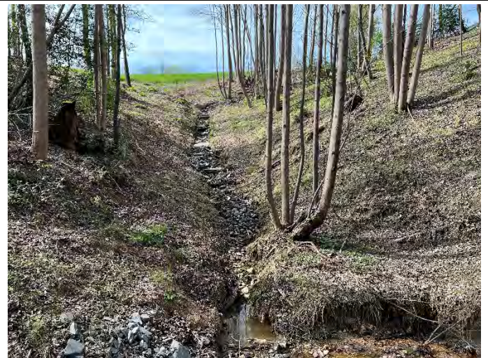
Upper UT1 repair area gully stabilization – 4/06/2022
