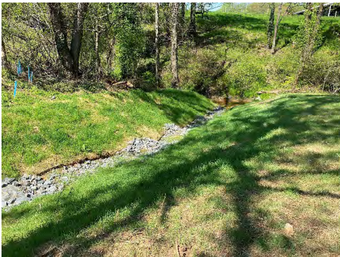
Silage Reach 1 STA 10+40 gully stabilization – 4/19/2021
