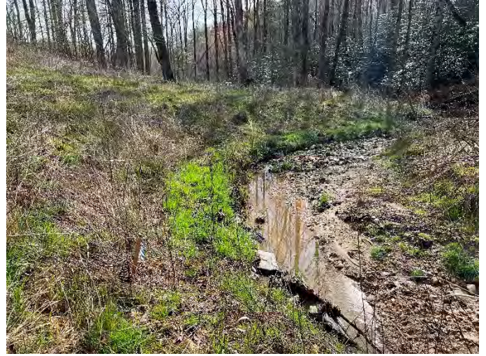
Silage Reach 1 STA 30+30 left bank repair – 4/06/2022
