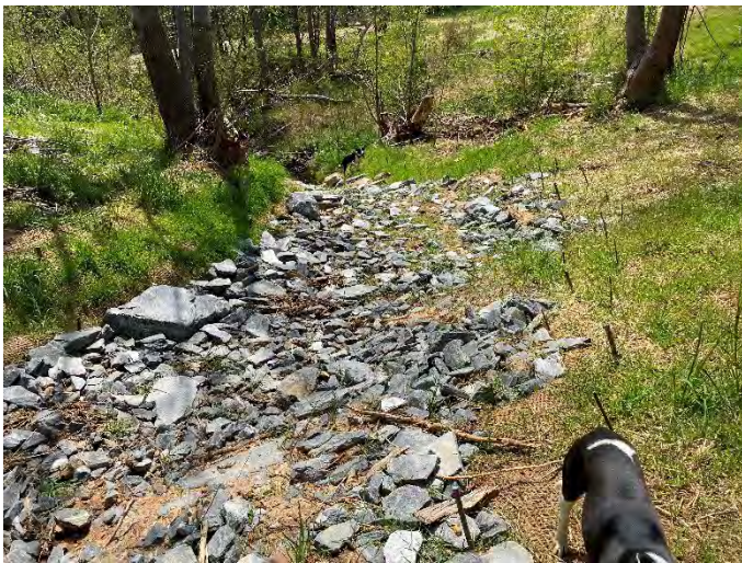
Upper Cow Trib 2 repair area – 4/20/2021
