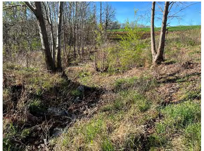
Upper Cow Trib 2 repair area – 4/06/2022
