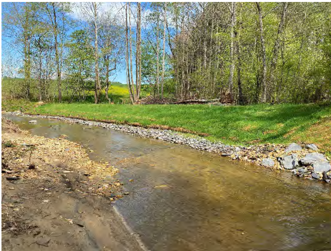
Moores Fork Reach 3 STA 64+10 left bank repair – 4/19/2021
