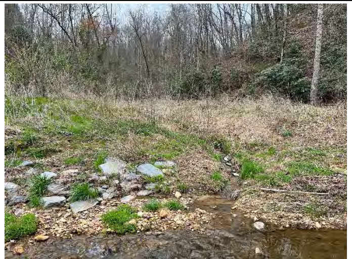
UT10/Wetland outlet repair at confluence with Moore's Fork – 4/05/2022
