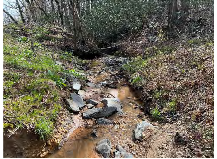
Silage Reach 1 STA 19+00 right bank repair – 4/06/2022
