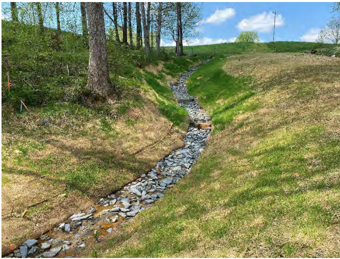
Upper Cow Trib 2 repair area gully stabilization – 4/20/2021
