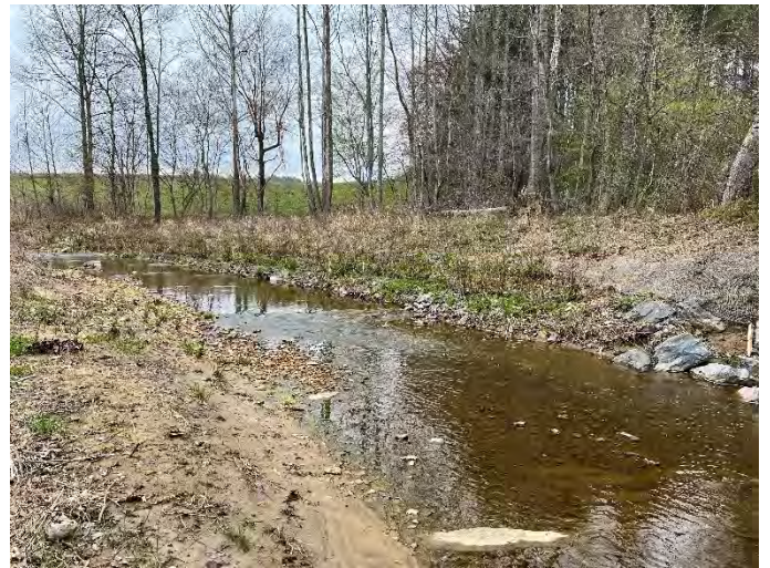
Moores Fork Reach 3 STA 64+10 left bank repair – 4/05/2022
