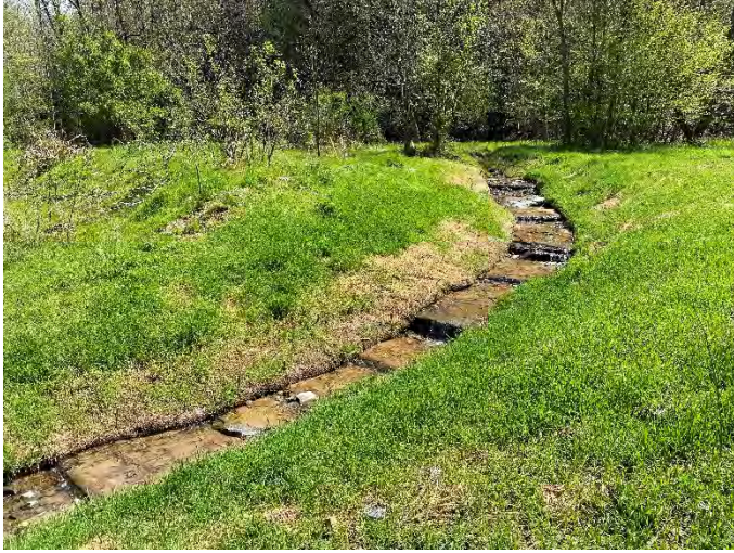
UT10/Wetland outlet repair – 4/19/2021
