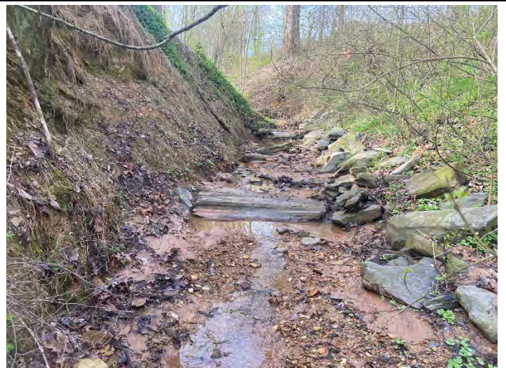
PP58 – Silage Reach 1, looking upstream (04/06/2022)
