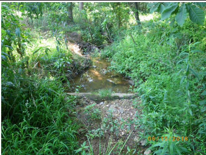
PP43 – Cow Tributary 2, looking downstream (06/15/2016)
