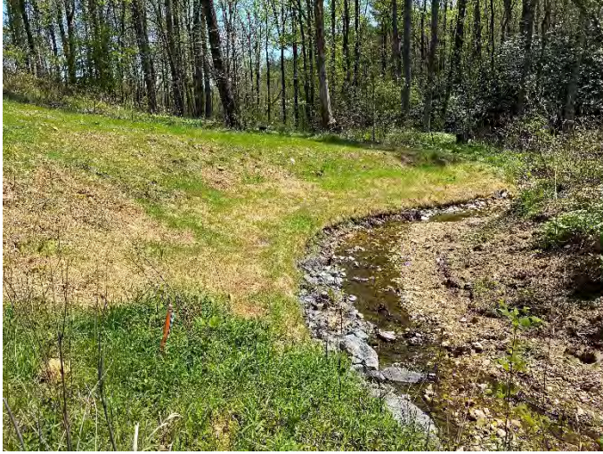
Silage Reach 1 STA 30+30 left bank repair – 4/20/2021
