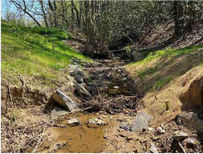
Silage Reach 1 STA 19+00 right bank repair – 4/20/2021
