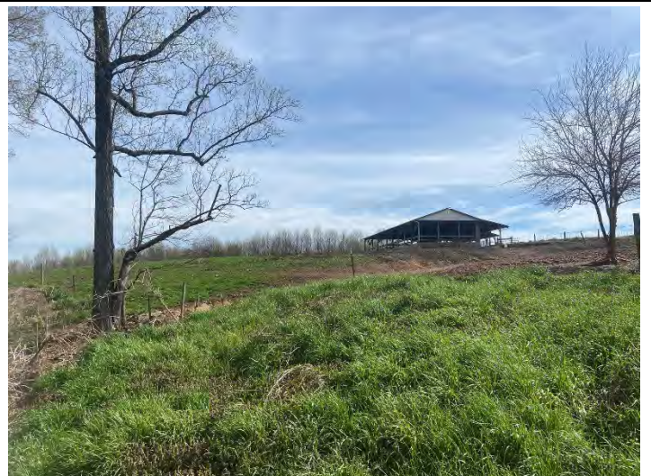
PP66 – Silage Reach 1, looking upslope (04/06/2022)
