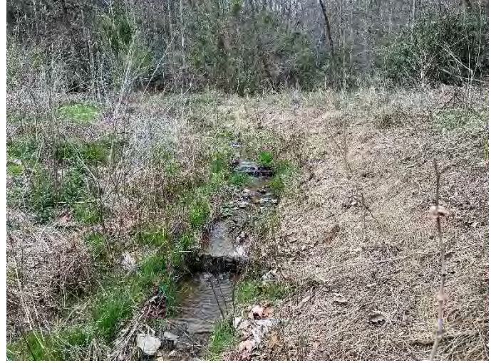
UT10/Wetland outlet repair – 4/05/2022
