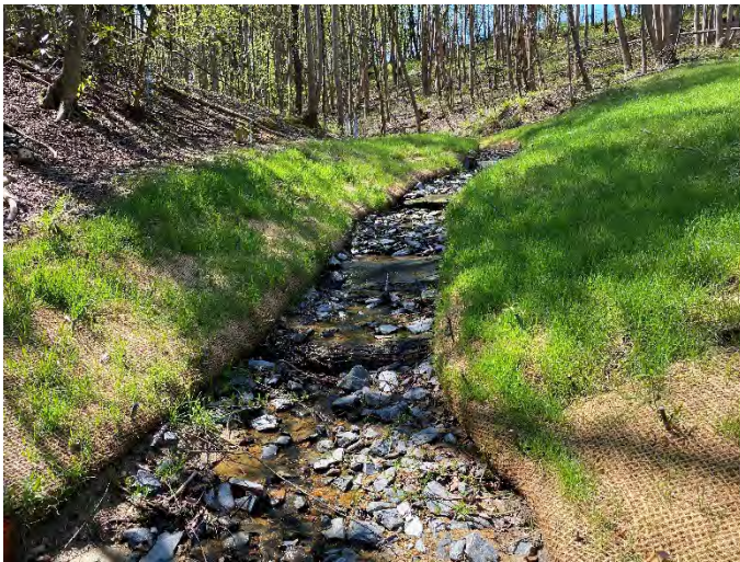
UT1 downstream repair near confluence with Silage Reach 1 – 4/20/2021
