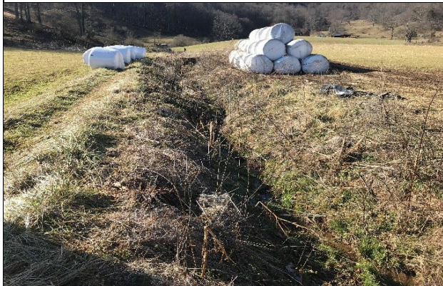
Photo 5: Channelized portion of T3. 1/24/2018
