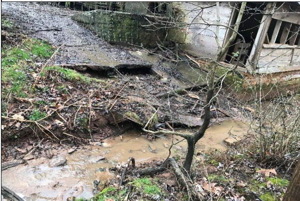
Photo 9: Cattle feed lot runoff spilling into T7. 1/24/2018
