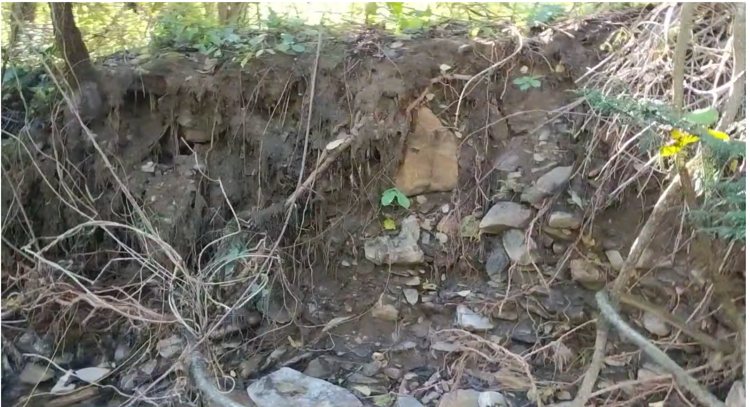
Formerly stable banks throughout this section are now unconsolidated and actively eroding after storm event requiring bank grading, stabilization, and bench grading (Area H).
