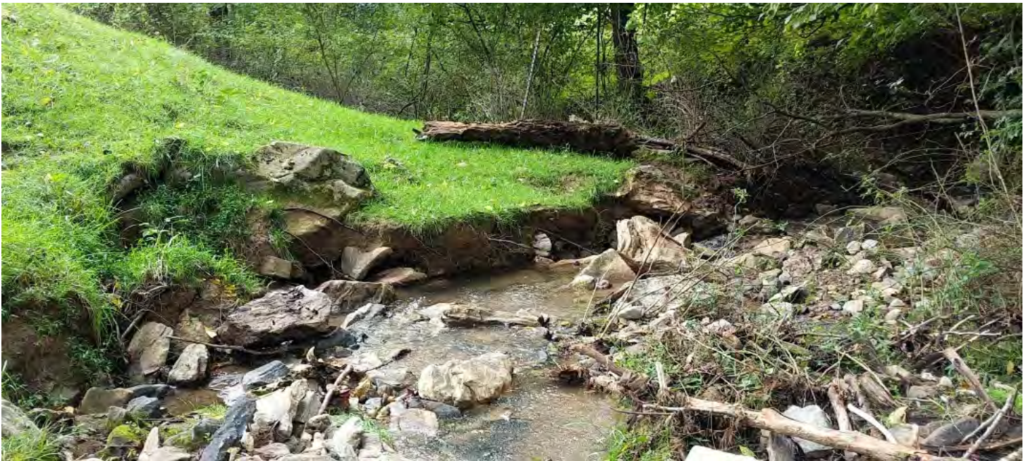
Another view on Morgan Branch of a formerly stable bank, now actively eroding after storm event requiring bank grading, stabilization, and bench grading (Area F).
