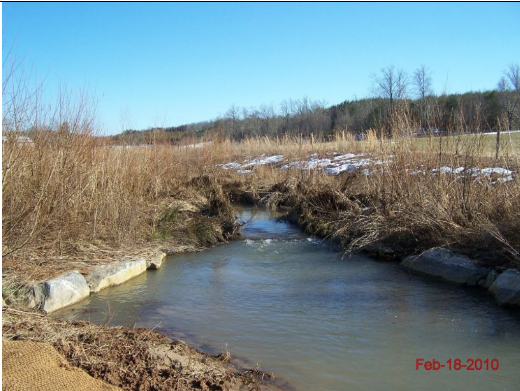
Permanent Photo Point #38 – Morgan Creek Looking Upstream
