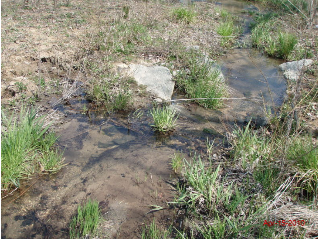
SPA2 UT1 Sta. 2001+50 – Grade Control Degradation
