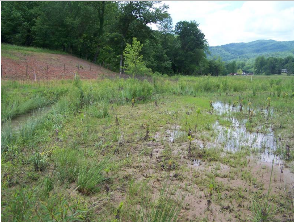
Wrack lines and deposition along Morgan Creek from bankfull event in May 2009
