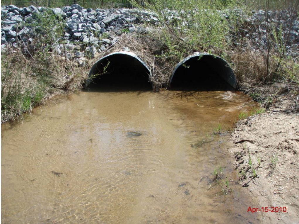
SPA4 Morgan Creek Sta. 1001+50 – Pool Aggradation
