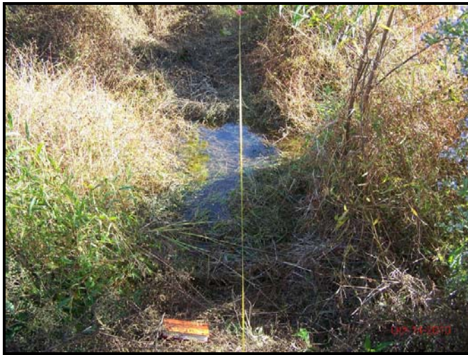
Looking at Left Bank
