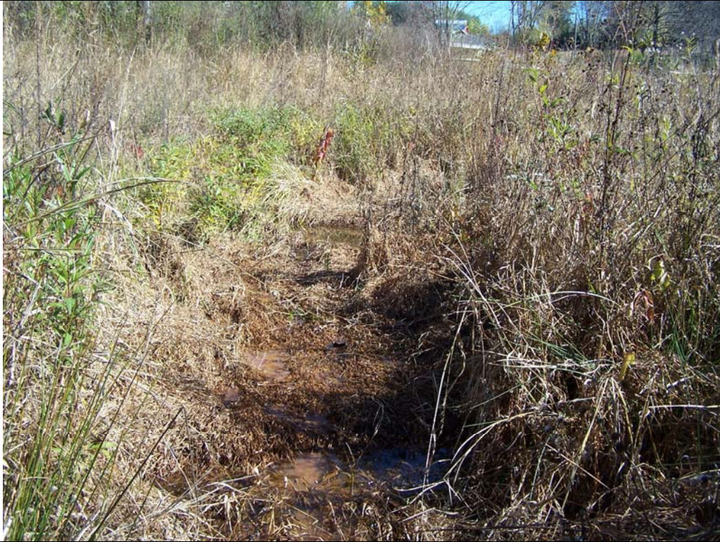
SPA 16 UT4 Sta. 5001+50 – Reduced pool depth and riffle fining due to aggradation November 11, 2010
