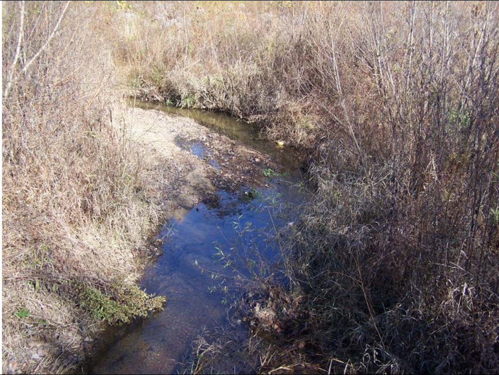
SPA 6 Morgan Creek Sta. 1001+50 – Reduced pool depth due to aggradation November 11, 2010
