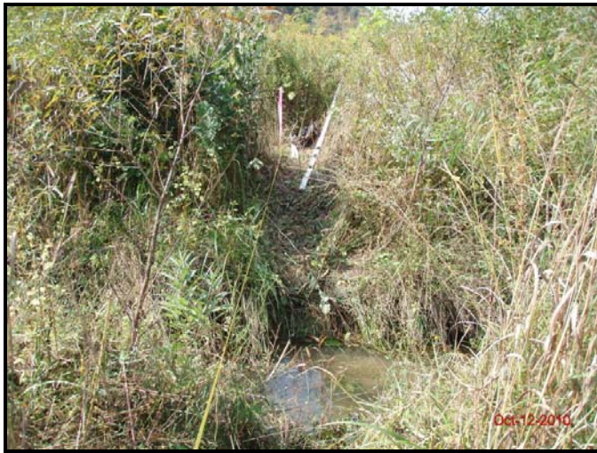
Looking at Left Bank
