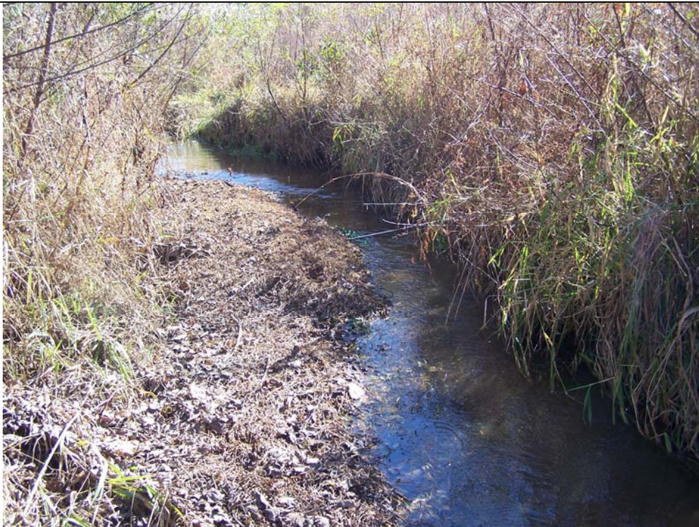
SPA 9 Morgan Creek Sta. 1003+25 – Reduced pool depth due to aggradation November 11, 2010
