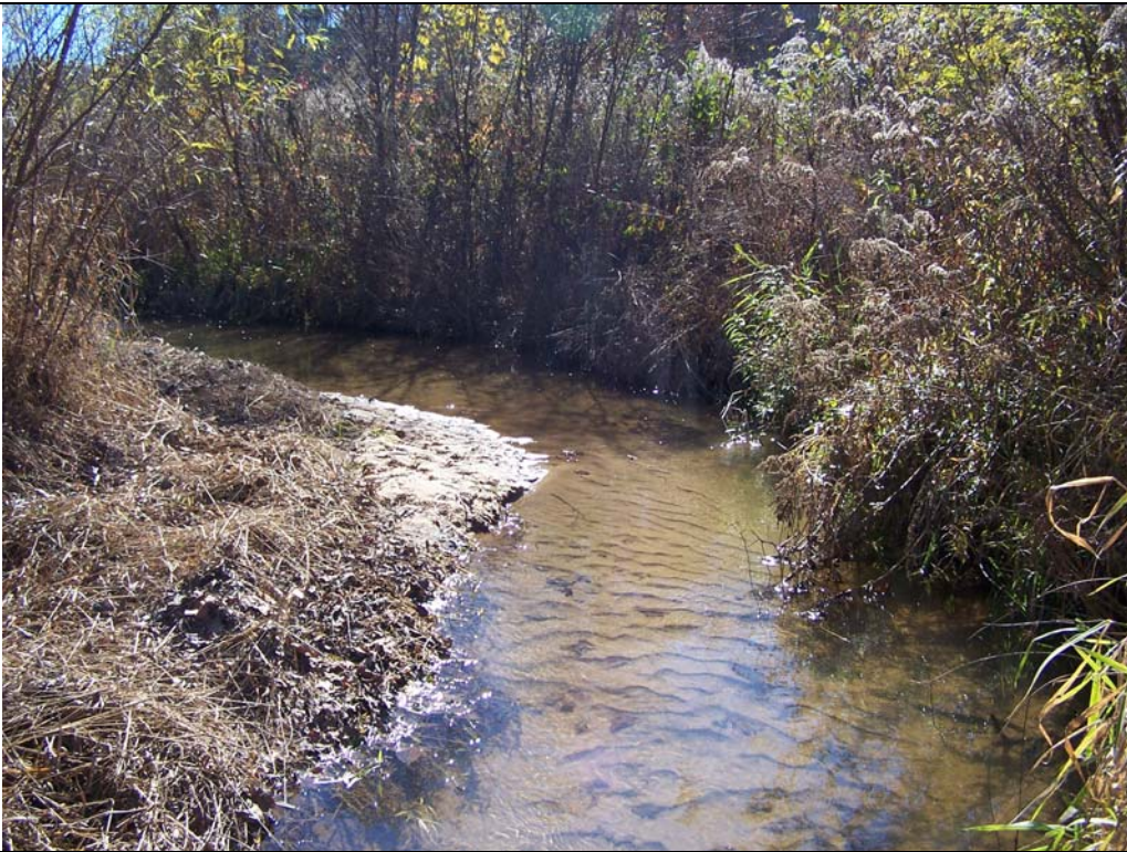
SPA 11 Morgan Creek Sta. 1005+05 – Reduced pool depth due to aggradation November 11, 2010
