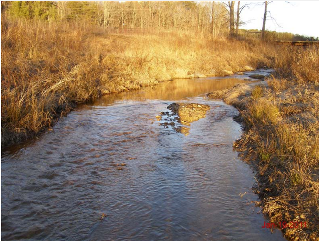
SPA 24 Morgan Creek Sta. 1047+00 – Reduced pool depth due to aggradation
