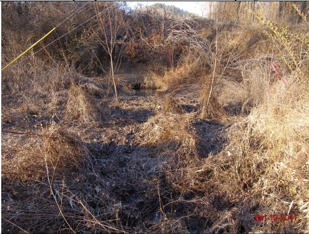
SPA 25 UT7 Sta. 8000+40 – Reduced pool depth and riffle fining due to aggradation
