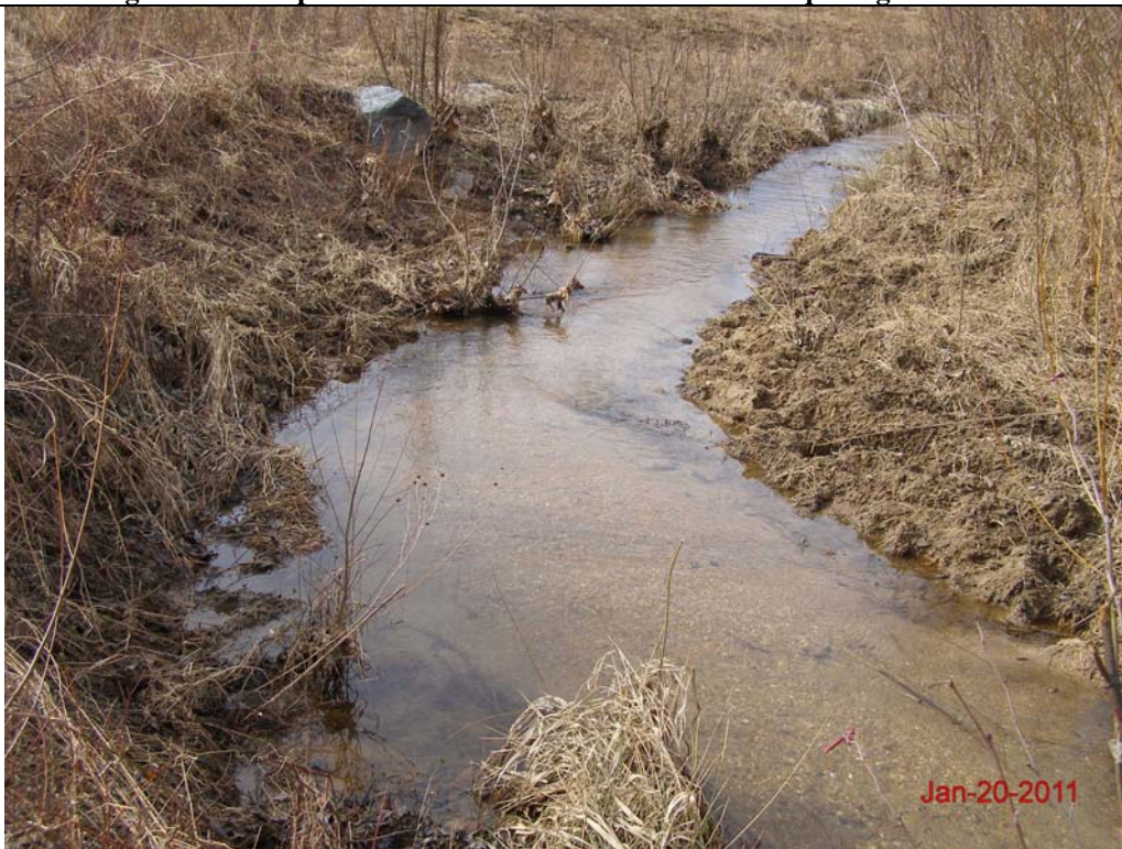
SPA 4 Morgan Creek Sta. 1002+25 – Reduced pool depth due to aggradation
