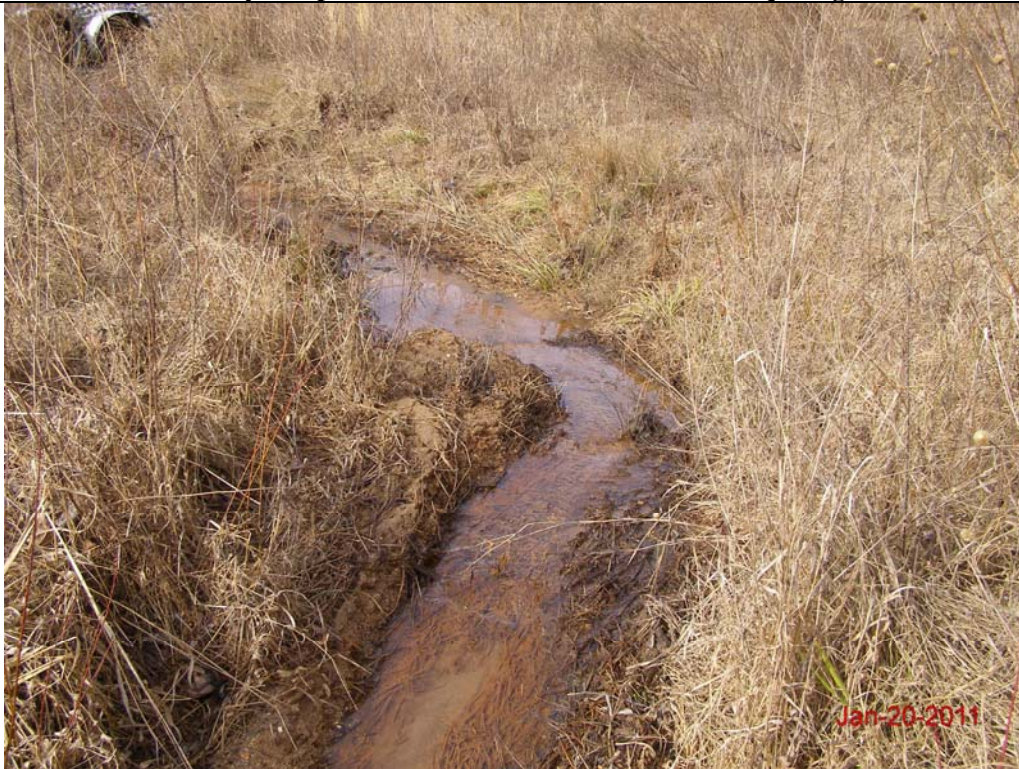
SPA 16 UT4 Sta. 5001+50 – Reduced pool depth and riffle fining due to aggradation
