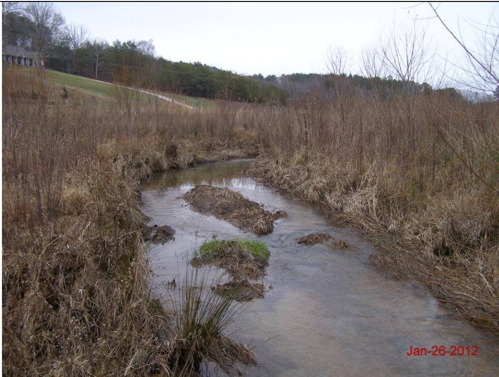
SPA 24 Morgan Creek Sta. 1038+50 – Reduced pool depth due to aggradation
