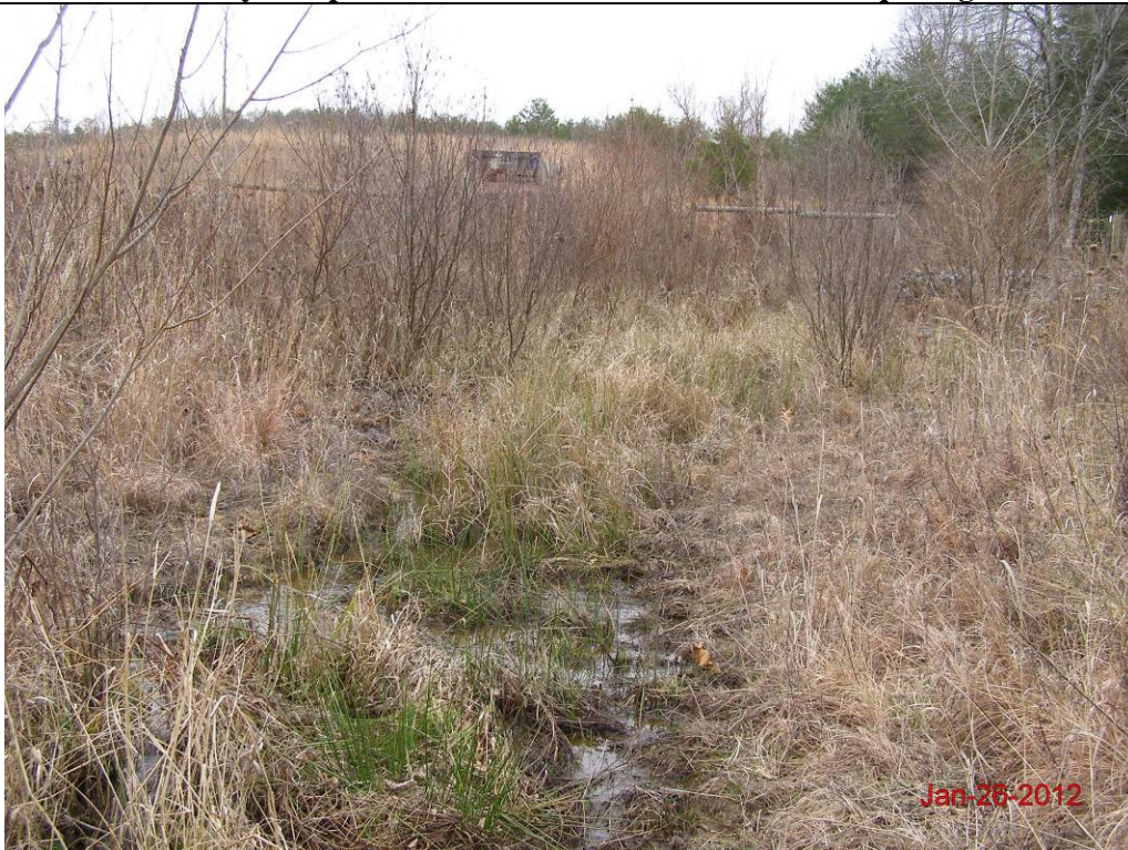
SPA 5 UT2 Sta. 3000+50 – Reduced pool depth and riffle fining due to aggradation
