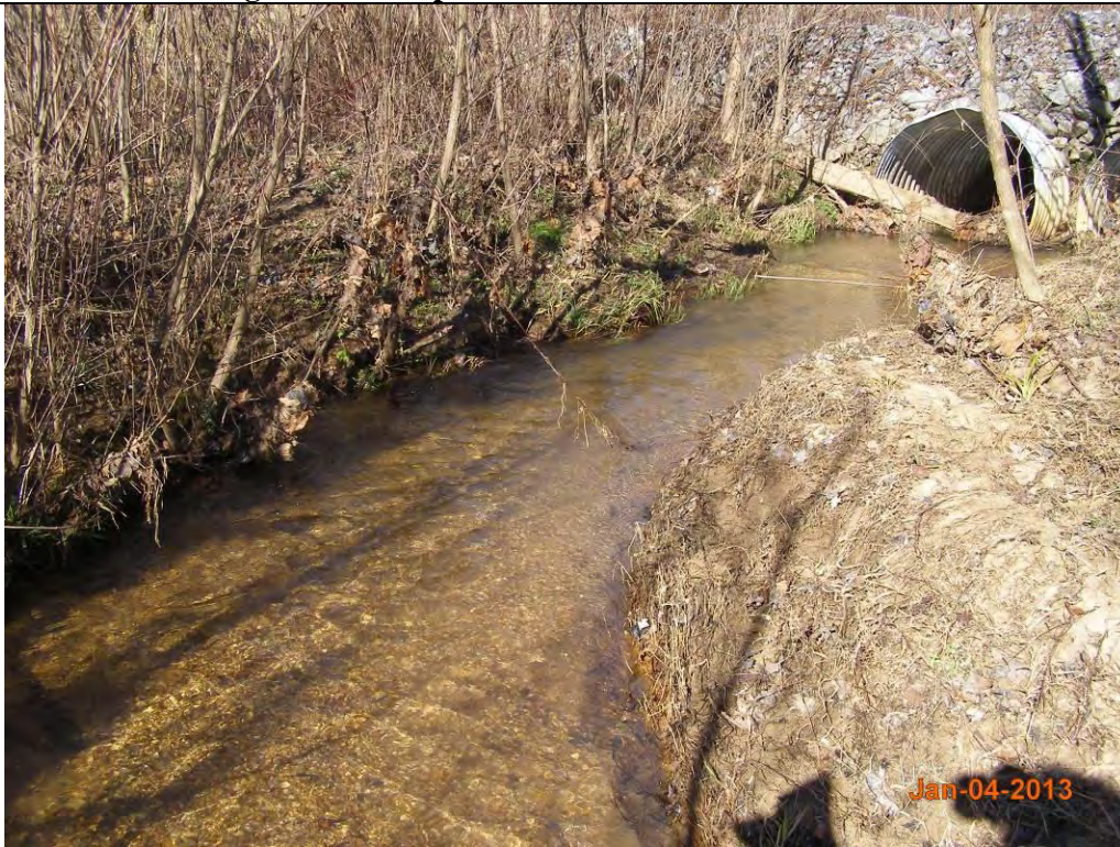
SPA 4 Morgan Creek Sta. 1003+25 – Reduced pool depth due to aggradation
