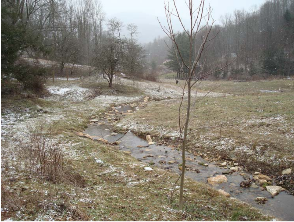
Morgan Creek facing downstream
