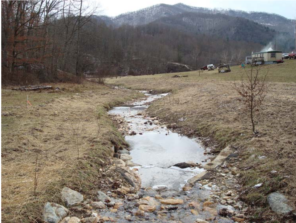
Piped crossing at easement break, facing downstream
