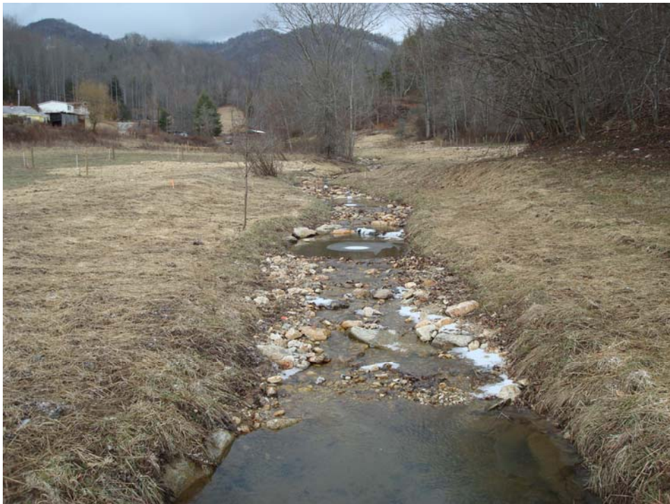
Piped crossing at easement break, facing upstream Photo No. 14
