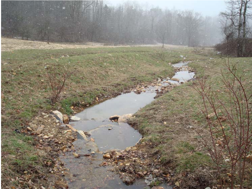
Lower North Branch from pipe outfall, facing downstream Photo No. 13
