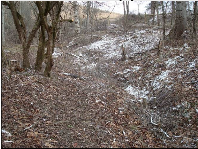
As-Built Photo No. 29 2/3/09
