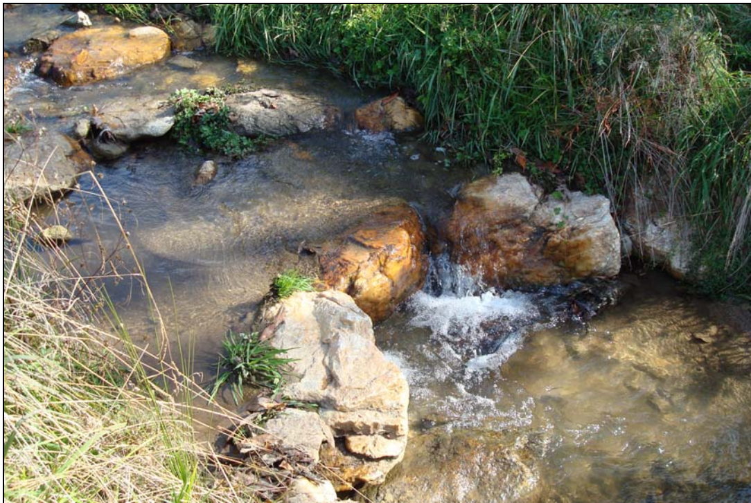
Excessive drop over structure, Morgan Cr, Sta 101+90 (Stable in Year 2) Year 1 10/30/09 Photo No. 16
