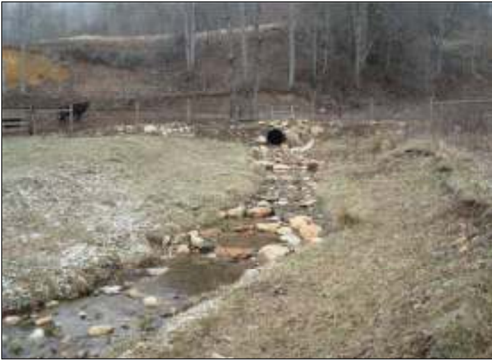
As-Built Photo No. 17 2/3/09
