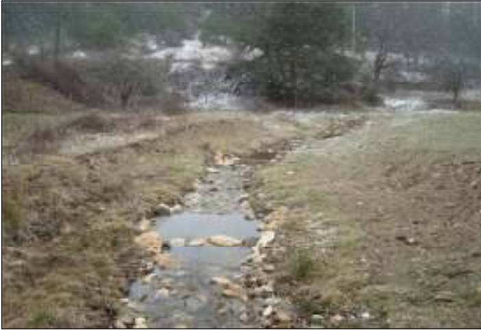
As-Built Photo No. 61 2/3/09
