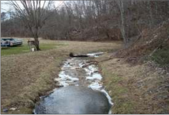
As-Built Photo No. 77 2/3/09
