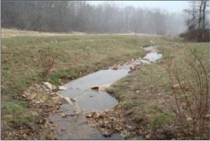
As-Built Photo No. 65 2/3/09
