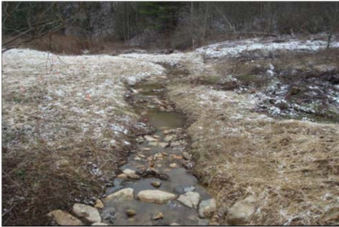
As-Built Photo No. 64 2/3/09
