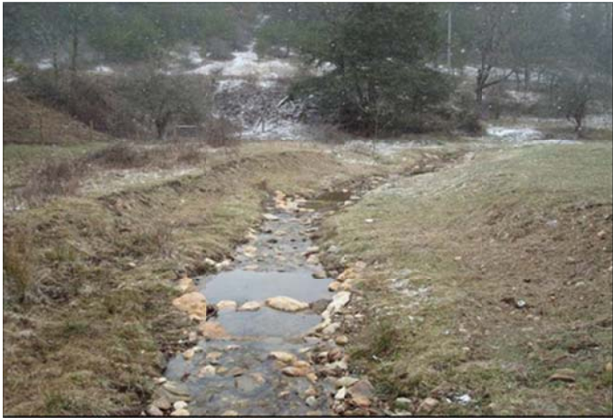
As-Built Photo No. 69 2/3/09
