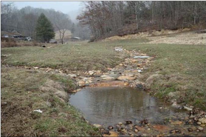
As-Built Photo No. 29 2/3/09
