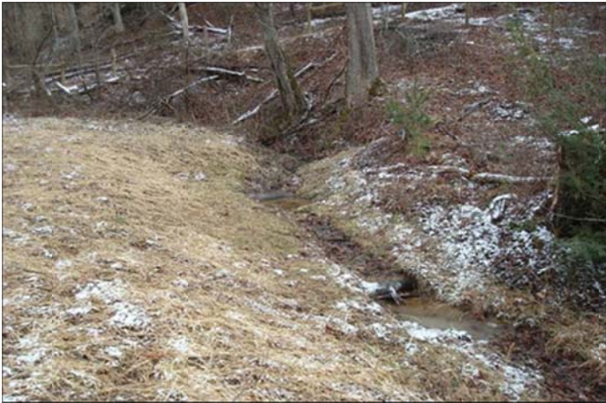
As-Built Photo No. 44 2/3/09
