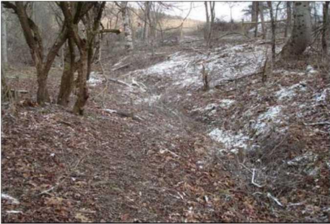
As-Built Photo No. 34 2/3/09
