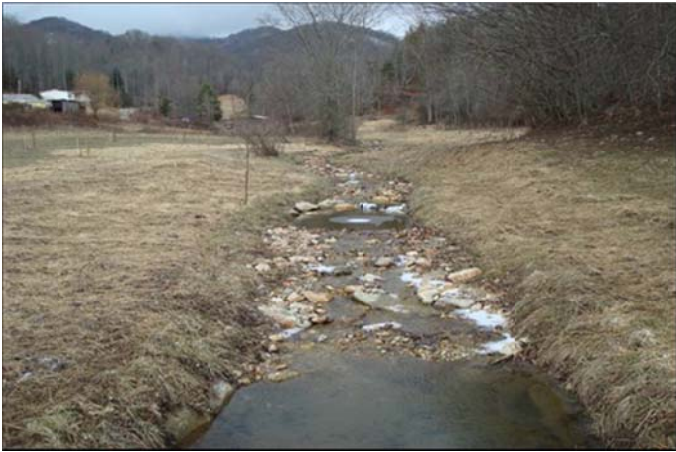
As-Built Photo No. 79 2/3/09
