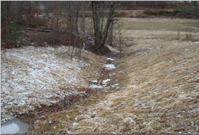
As-Built Photo No. 49 2/3/09
