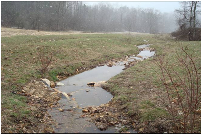
As-Built Photo No. 79 2/3/09
