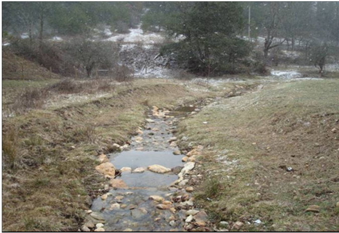
As-Built Photo No. 73 2/3/09
