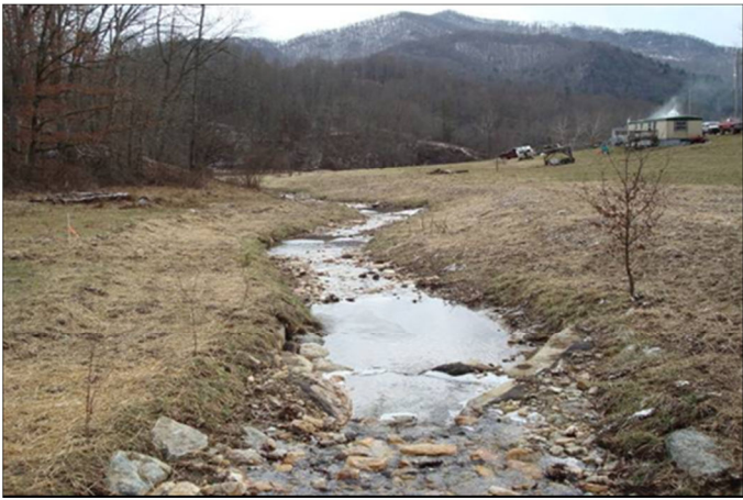
As-Built Photo No. 91 2/3/09
