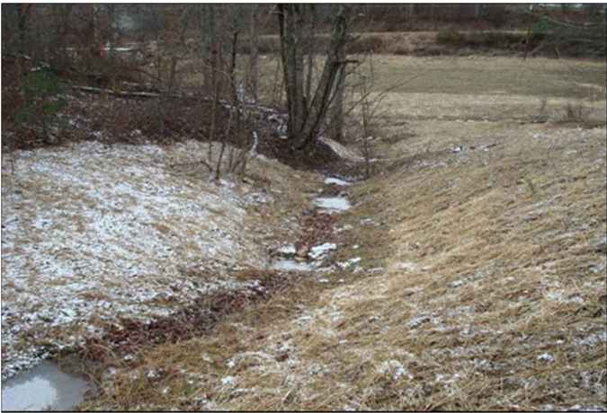
As-Built Photo No. 49 2/3/09
