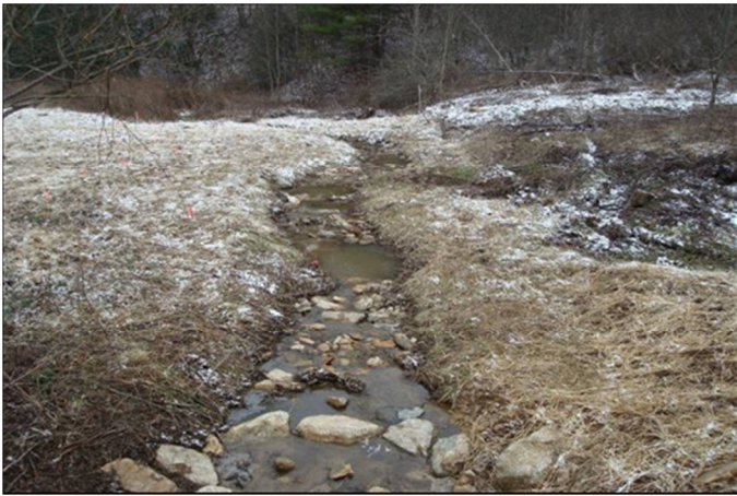
As-Built Photo No. 67 2/3/09
