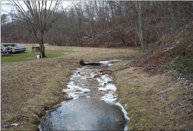
As-Built Photo No. 97 2/3/09
