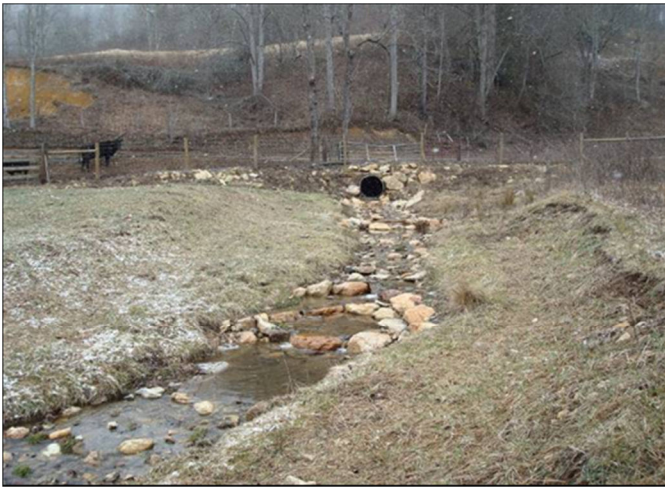
As-Built Photo No. 13 2/3/09
