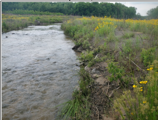
SPA3 – Localized scour along left bank from eddying within the riffle (looking upstream)
