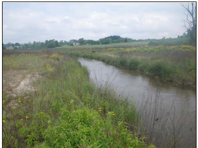
South Muddy Creek PID 18 – Constructed Riffle
