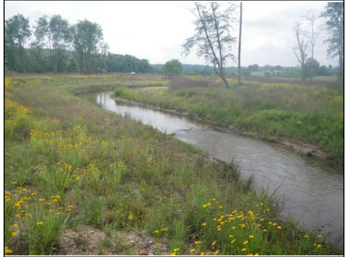
South Muddy Creek PID 20 – J-Hook near downstream end of project
