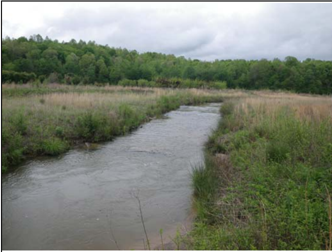
South Muddy Creek PID 13 – Constructed Riffle
