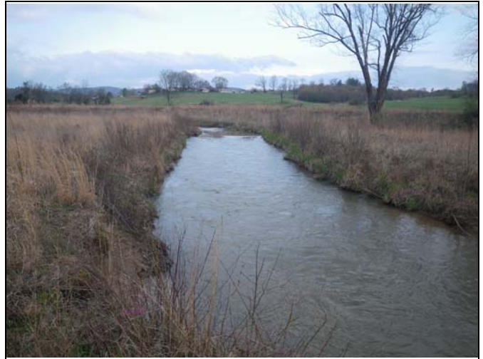
South Muddy Creek PID 8 – Constructed Riffle
