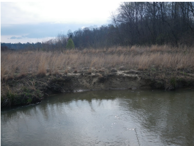
SPA2-3 – Localized scour along right bank within a riffle from the lack of thalweg centering downstream of a meander bend (looking across from left to right bank)
