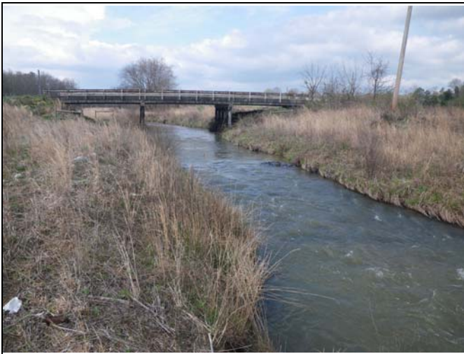
South Muddy Creek PID 15 – Constructed Riffle downstream of Sain Road crossing
