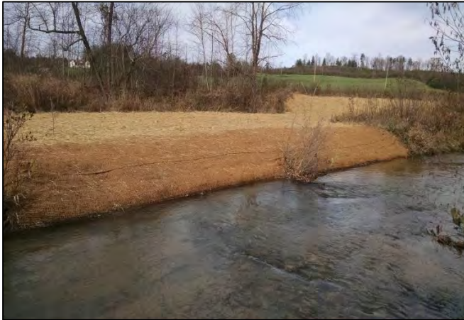
Downstream photo of bank repair completed in November 2015.
