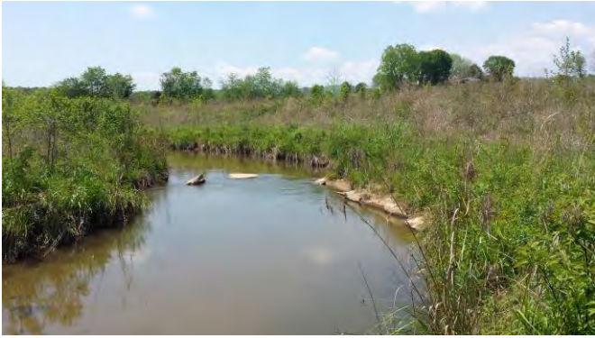
South Muddy Creek PID 7 – J-Hook in Meander
