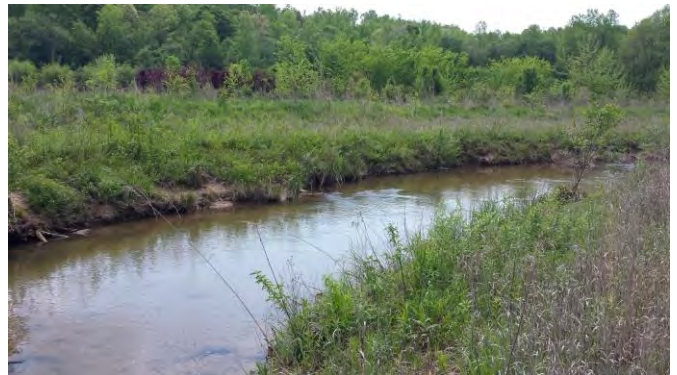
South Muddy Creek PID 12 – Log Vane and Root Wad in Meander
