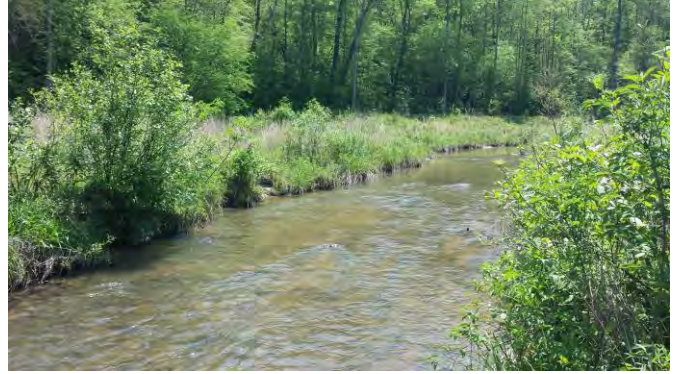
South Muddy Creek PID 2 –Constructed Riffle,
