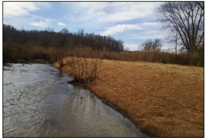
Upstream photo of bank repair completed in November 2015.
