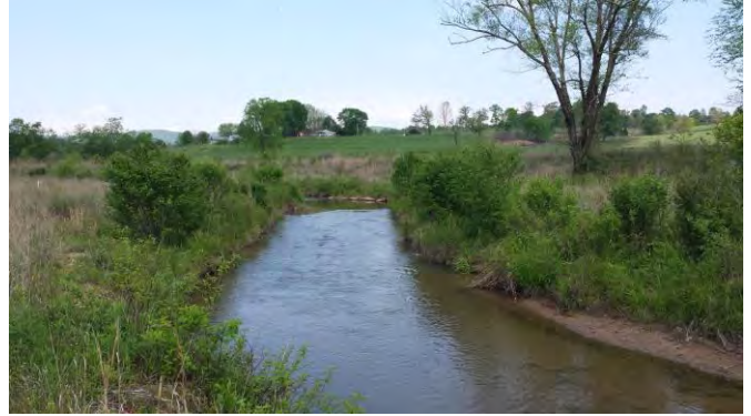
South Muddy Creek PID 8 – Constructed Riffle
