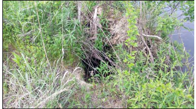
SPA4-2 – Localized scour along right bank behind rootwads (looking downstream from right bank). Possibly caused by animals.
