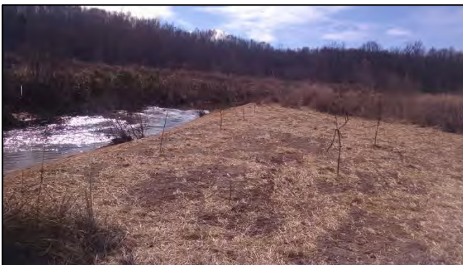
Floodplain view of repair area and plantings.
