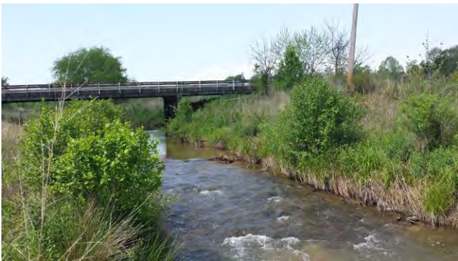
South Muddy Creek PID 15 – Constructed Riffle downstream of Sain Road crossing
