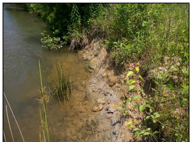
SPA3-2 – Localized scour along right bank downstream of Sain Rd. Bridge (5-25-26).
