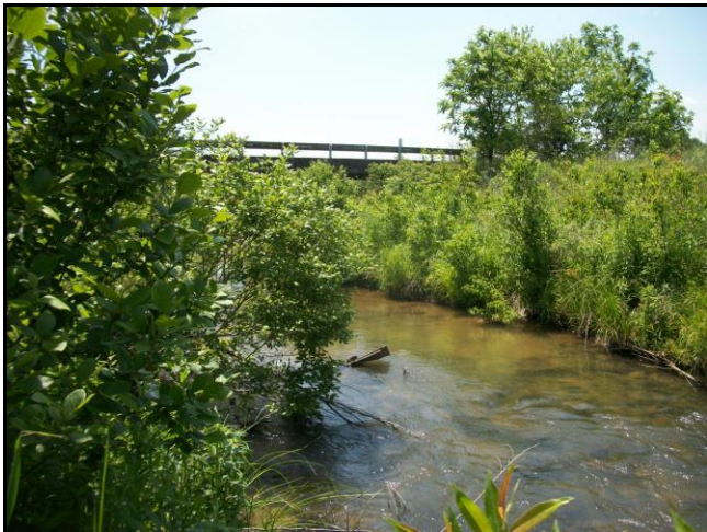
South Muddy Creek PID 15 – Constructed Riffle downstream of Sain Road crossing
