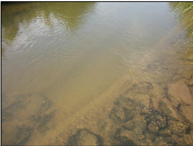
SPA5-2 – Scour from SPA4-1 has led to structure failure of both the rootwad and the log sill. The root wad is no longer functioning and has separated from bank; however, it still seems to be tied into the bank. The log sill has separated completely from the bank and is now resting entirely upon the bed of the channel (5-26-16).
