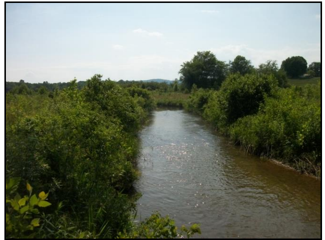
South Muddy Creek PID 4 – Constructed Riffle
