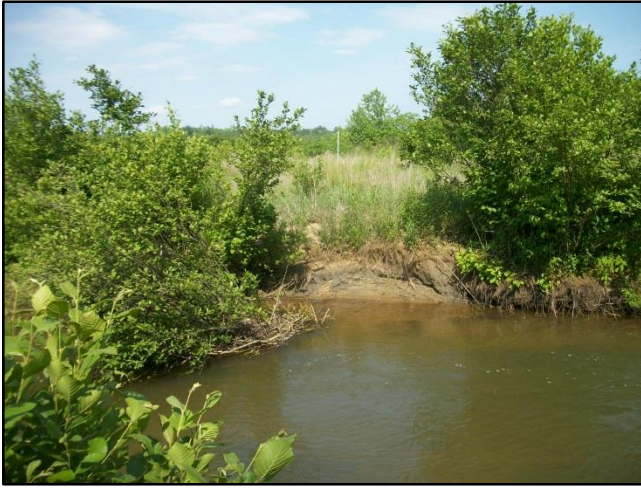
SPA 5-4 – Scour pocket causing a loss of stream bank vegetation on the right bank along the inside of the meander bend (5-25-16)
