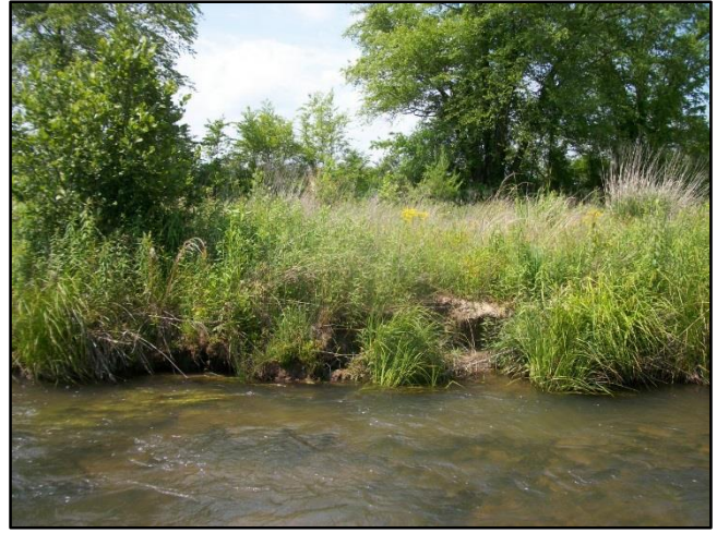
SPA 5-5 – Scour and bank slumping along left bank (5-25-16)
