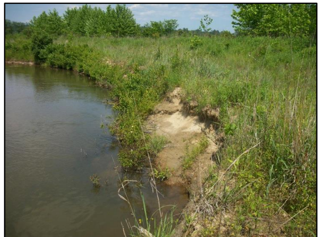
SPA 5-3 – Scour pocket on right bank just downstream of rock j-hook boulder tie-in has caused the boulder/bank tie-in to be breached (5-25-16)
