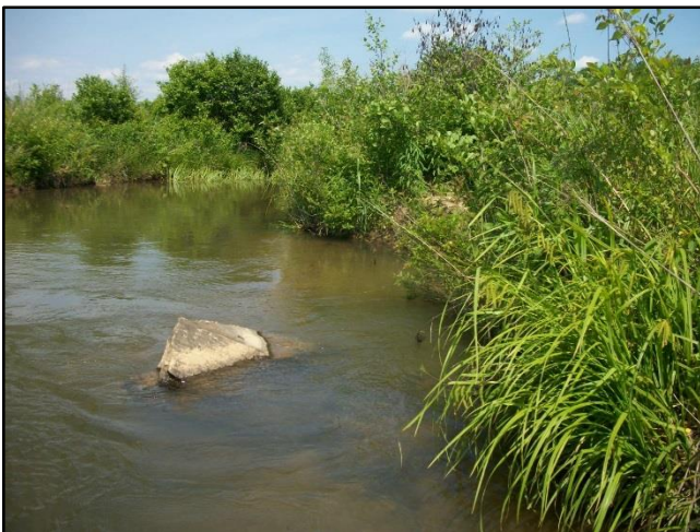
SPA 5-3 – Scour pocket on right bank just downstream of rock j-hook boulder tie-in has caused the boulder/bank tie-in to be breached (5-25-16)
