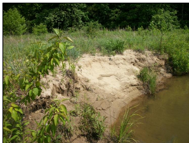
SPA2-3 – Localized scour along right bank along riffle from the lack of thalweg re-centering (5-25-16).
