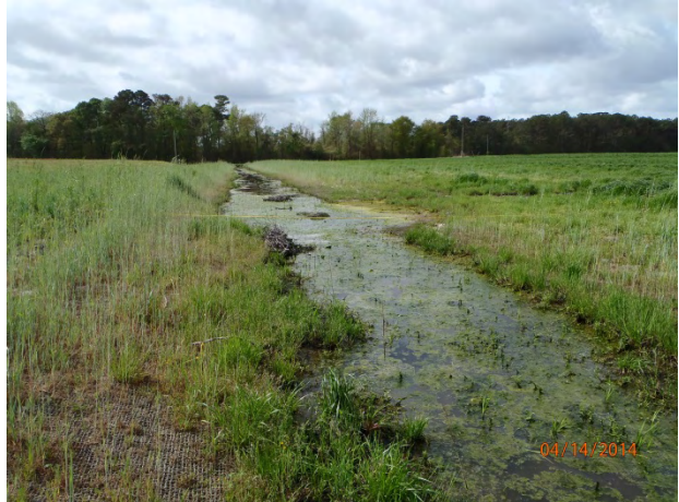
Reach 1A HWV – Looking Downstream - Sta. 2+80 Post-Construction (04/14/2014)
