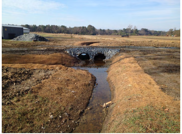
Reach 1B Looking Downstream Sta. 34+00 - Crossing (12/03/2013)
