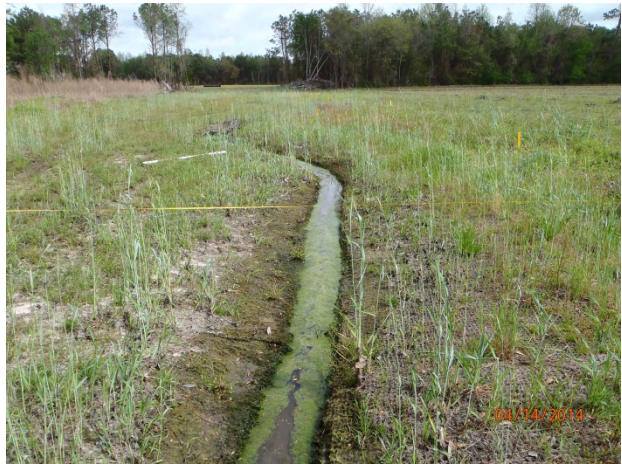
Reach 1A Looking Downstream Sta. 14+80 – Post-Construction (04/14/2014)
