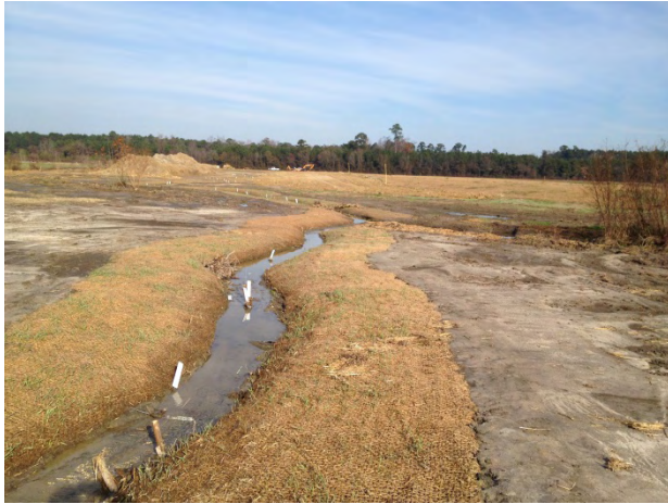
Reach 2 Looking Downstream Sta. 8+15 - Post-Construction (12/03/2013)
