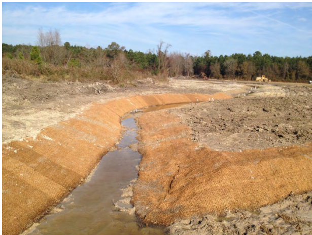
Reach 1C/3 Looking Upstream Sta. 47+80 - Confluence (12/03/2013)
