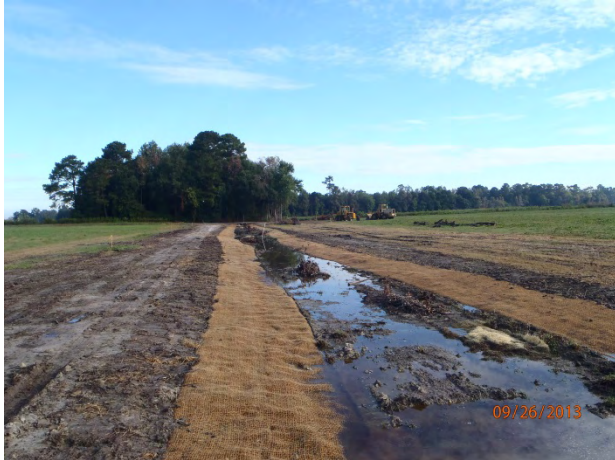
Reach 1A HWV – Looking Downstream - Sta. 2+80 Construction (09/26/2013)
