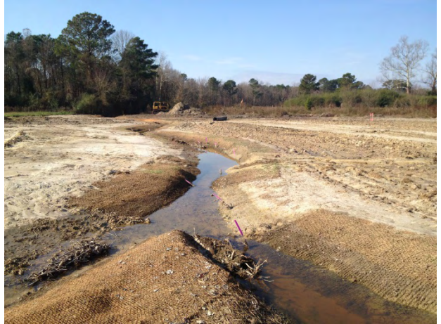
Reach 1C/2 Looking Downstream Sta. 45+50 - Confluence (12/03/2013)
