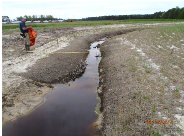
Reach 3 Looking Downstream Sta. 3+20 -Post-Construction (04/14/2014)
