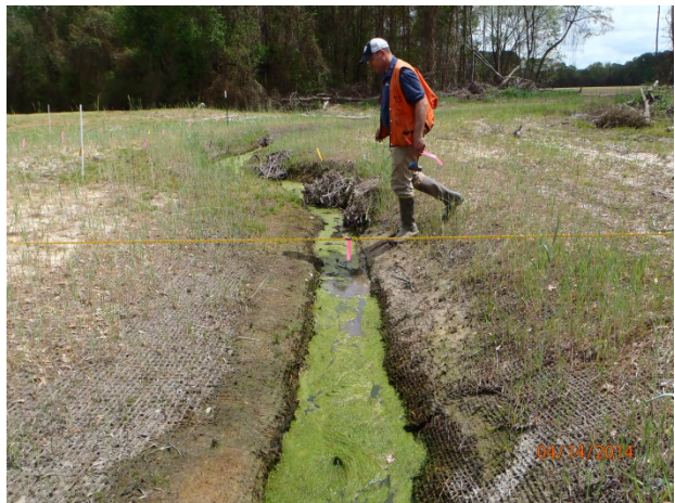
Reach 1A Looking Downstream Sta. 20+55 – Post-Construction (04/14/2014)
