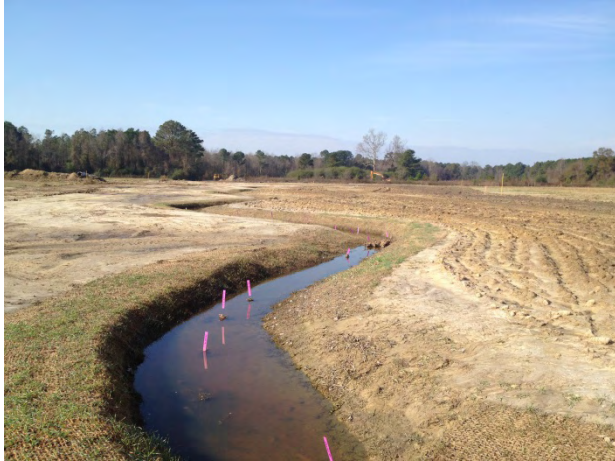
Reach 1C Looking Downstream Sta. 39+50 - Post - Construction (12/03/2013)
