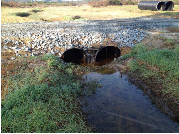
Reach 1A/1B Looking Downstream Sta. 22+00 - Crossing (12/03/2013)
