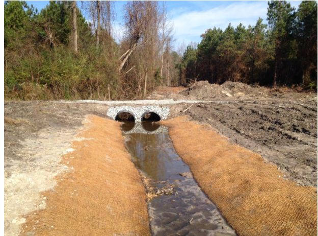
Reach 3 Looking Upstream Sta. 1+50 - Crossing (12/03/2013)
