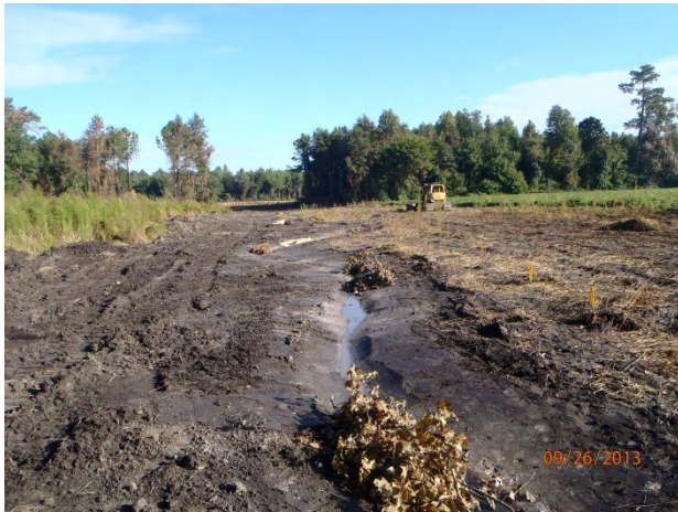
Reach 1A Looking Downstream Sta. 14+80 - Construction (09/26/2013)
