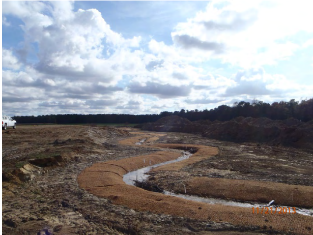
Reach 2 Looking Upstream Sta. 16+10 - Construction (11/21/2013)
