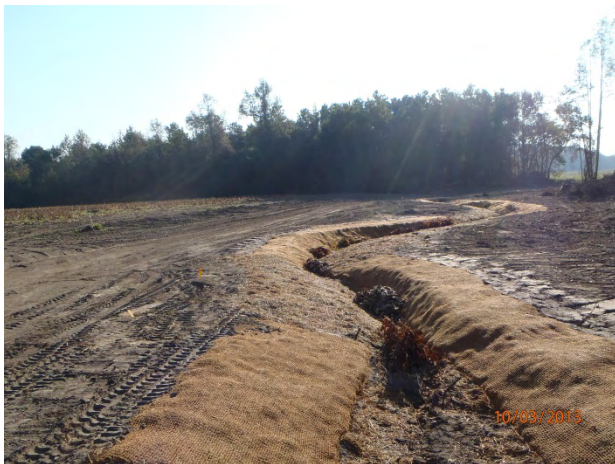
Reach 1A Looking Downstream Sta. 20+55 - Construction (10/03/2013)
