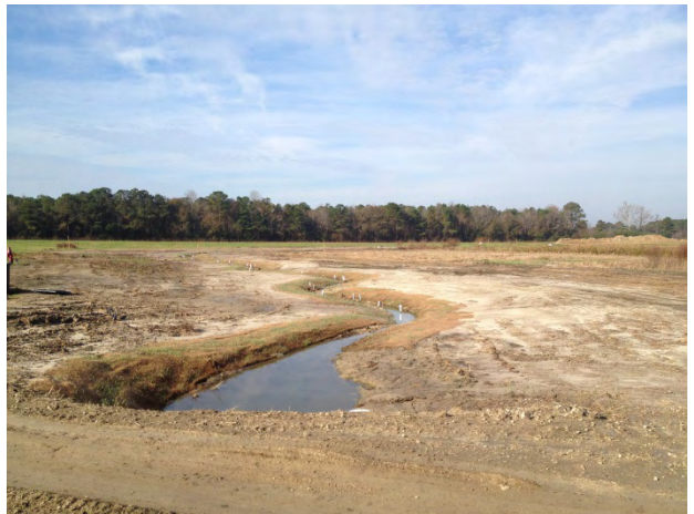
Reach 2 Looking Downstream Sta. 2+00 - Post - Construction (12/03/2013)
