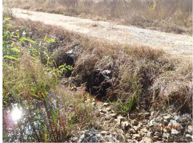
Reach 1B/1C Looking Downstream Sta. 34+00 - Crossing- MY1 (11/12/2014)
