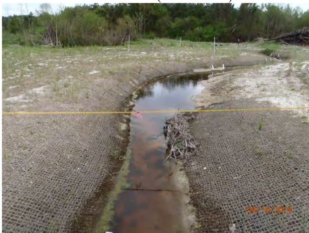
Reach 3 Looking Upstream Sta. 2+50 - Post-Construction (04/14/2014)
