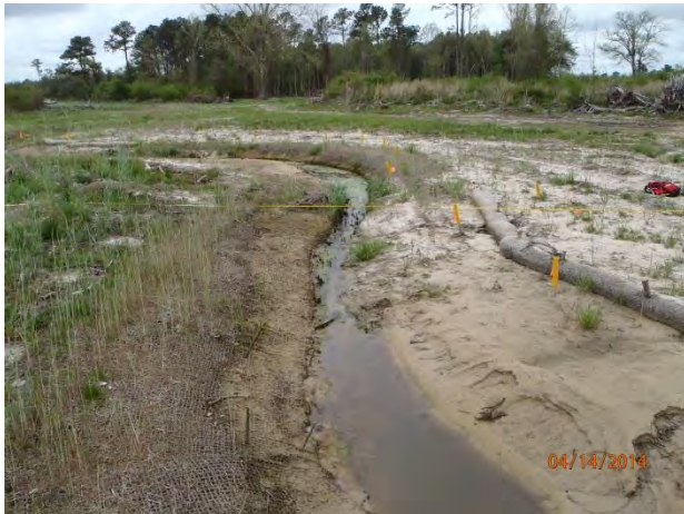
Reach 1B Looking Downstream Sta. 26+50 - Post-Construction (04/14/2014)
