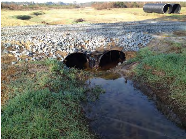
Reach 1B Looking Downstream Sta. 22+00 - Crossing (12/03/2013)
