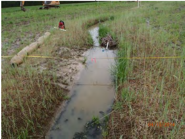
Reach 2 Looking Downstream Sta 5+20- Post-Construction (04/15/2014)
