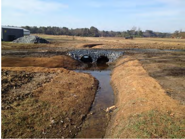
Reach 1B/1C Looking Downstream Sta. 34+00 - Crossing (12/03/2013)
