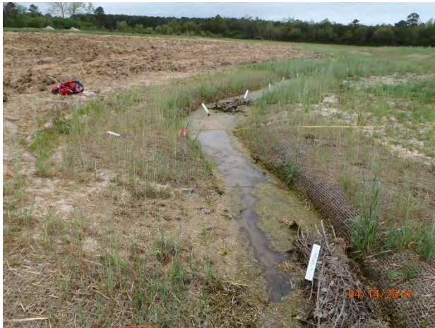
Reach 2 Looking Downstream Sta. 11+50 - Post-Construction (04/14/2014)
