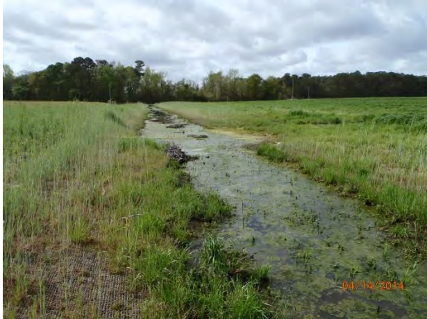
Reach 1A HWV – Looking Downstream - Sta. 2+80 Post- Construction (04/14/2014)
