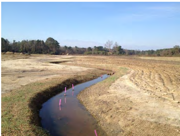
Reach 1C Looking Downstream Sta. 39+50 - Post-Construction (12/03/2013)
