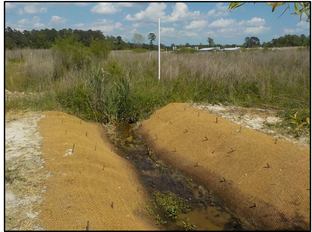
MY2-SP2 Minor Bed Erosion at Sta 47+15 - 47+45. (Repaired in April 2016)
