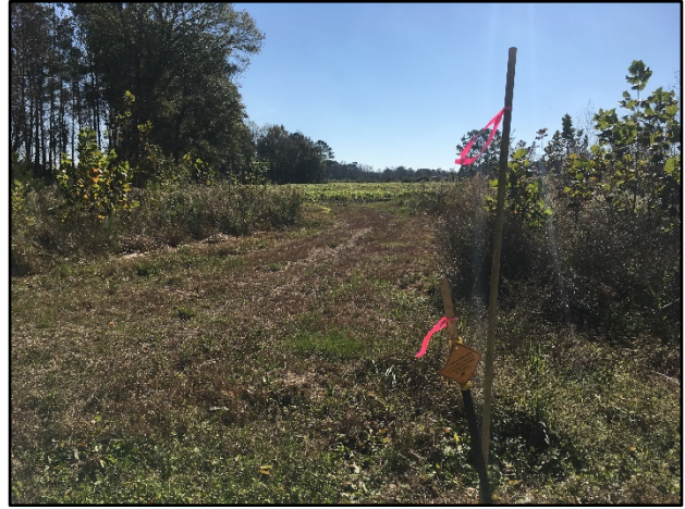
MY4-VPA1 Encroachment at Reach 1B Sta 21+50
