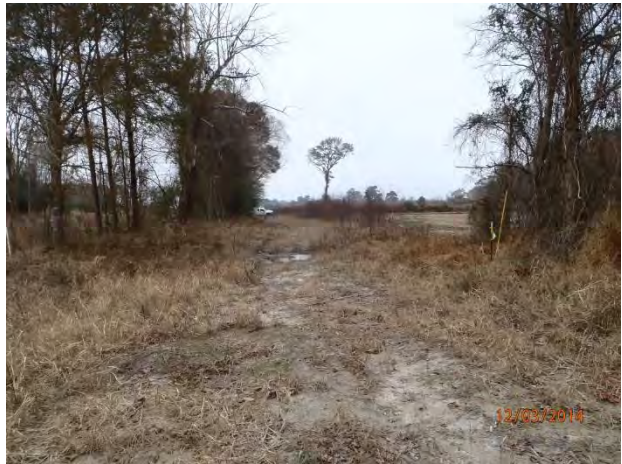
VPA4- Missing rows of trees and vehicles through easement along Reach 3a @ Sta 19+00 - Sta 23+00
