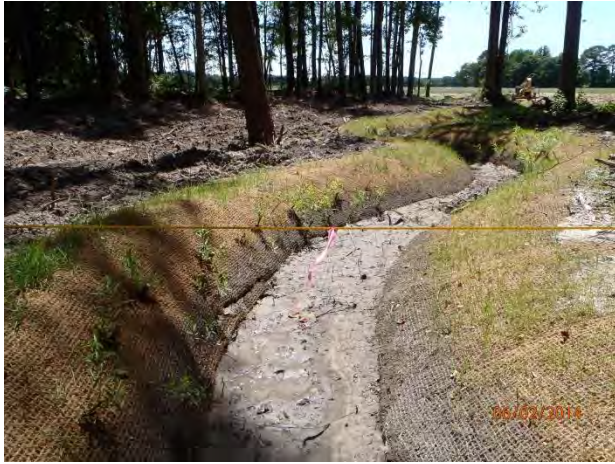
Reach 2 Looking Downstream Sta. 16+35 Post-Construction (05/22/2014)
