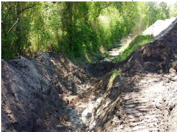
Reach 5B Looking Downstream Sta. 20+05 During Construction (04/23/2014)
