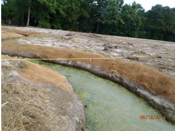
Reach 5A Looking Downstream Sta. 17+80 Post-Construction (06/18/2014)
