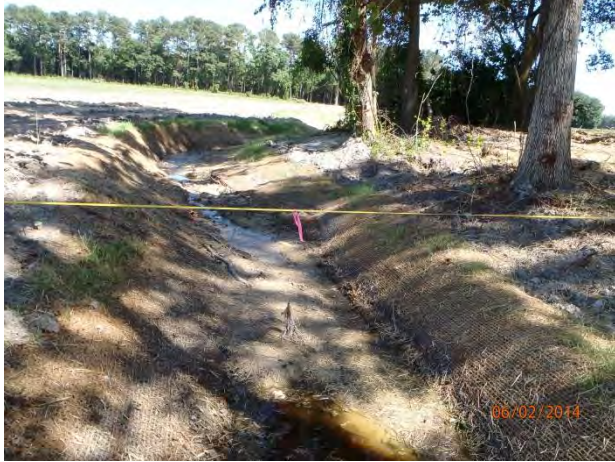
Reach 3A Looking Downstream Sta. 7+50 During Construction (06/02/2014)
