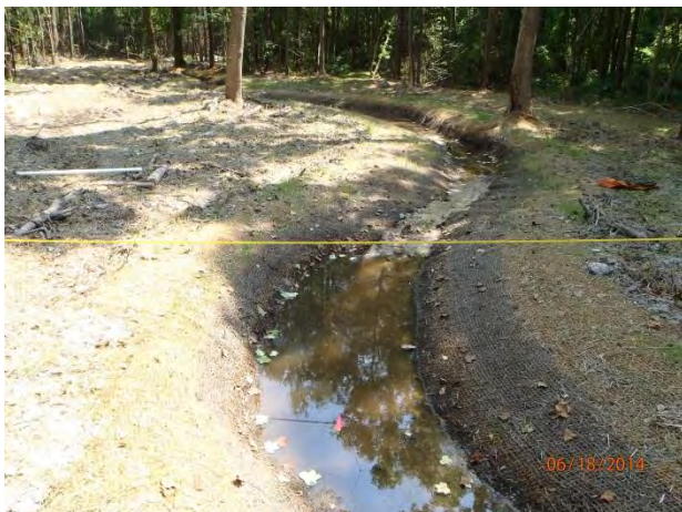
Reach 3B Looking Upstream Sta. 48+70 Post-Construction (06/18/2014)
