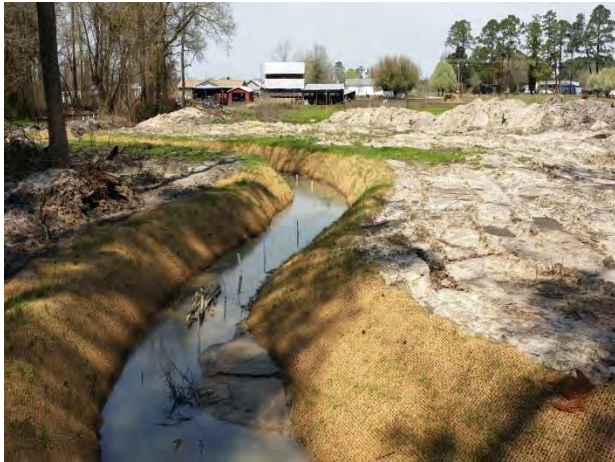
Reach 3B Sta. 44+75 Looking Downstream During Construction (04/03/2014)
