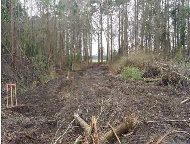
Reach 6 Looking downstream Sta. 8+00 During Construction (03/12/2014)
