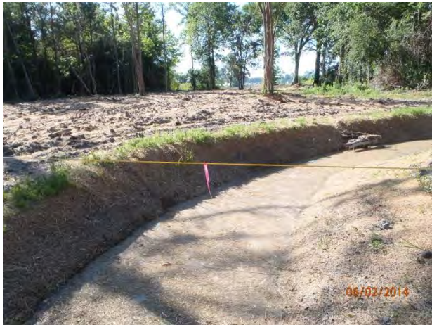
Reach 3A Looking Downstream Sta. 19+80 Post-Construction (06/02/2014)
