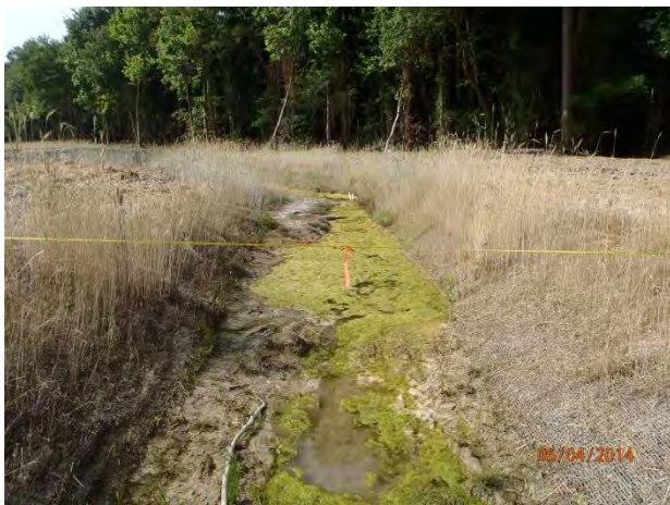
Reach 5a Looking Upstream Sta. 13+50- Post Construction (06/04/2014)
