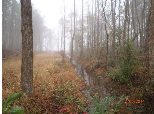
Reach 6 Looking downstream Sta. 8+00- MY1 During Construction (12/03/2014)
