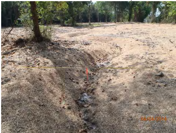
Reach 4 Looking Downstream Sta. 0+65- Post Construction (06/02/2014)
