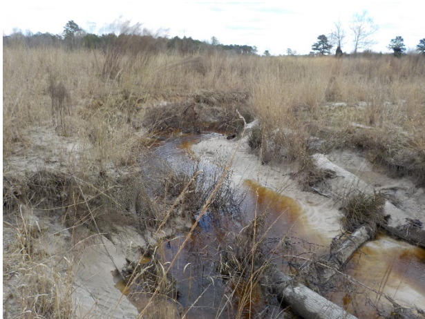
SPA5- Failed grade control structures and bank erosion- Reach 5A @ Sta 13+25- Sta 16+50
