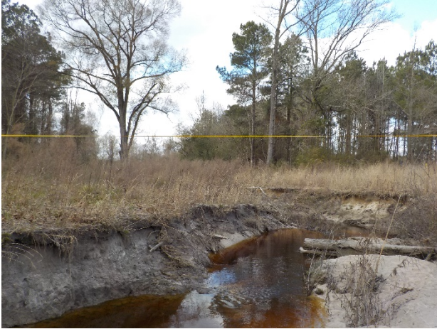
SPA5- Failed grade control structures, bed/bank erosion- Reach 5A @ Sta 16+50- 19+50
