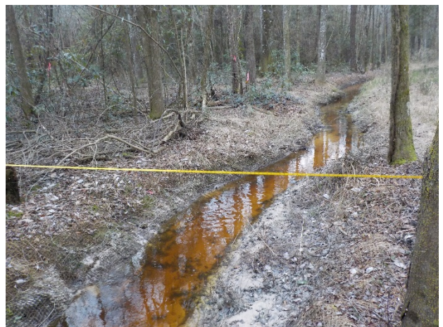
Reach 3B Looking Downstream Sta. 52+25-MY2 (2/10/2016)
