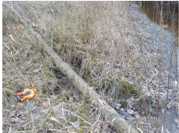
SPA4- Minor left bank erosion – Reach 3C @ Sta 60+00 and 61+00
