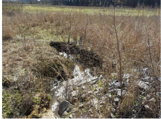
SPA2- Left bank erosion behind flow diversion structure - Reach 3b @ Sta 37+22
