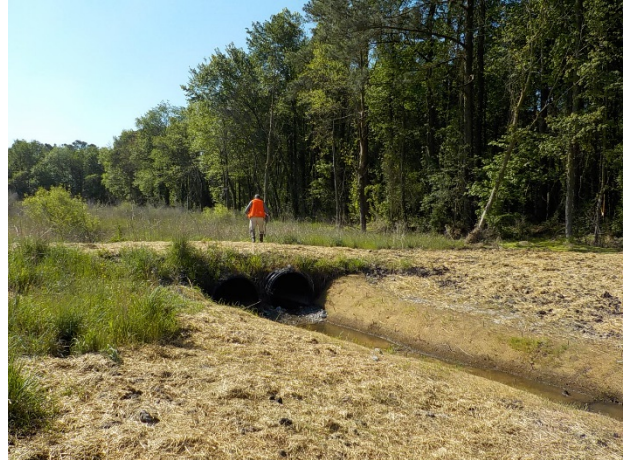
SPA5-MY2-2015 Reach 5A Repairs (4/26/2016)
