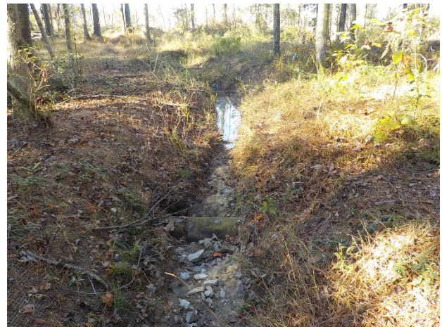
SPA2-MY2-2015 Repaired Structures (11/8/2016)
