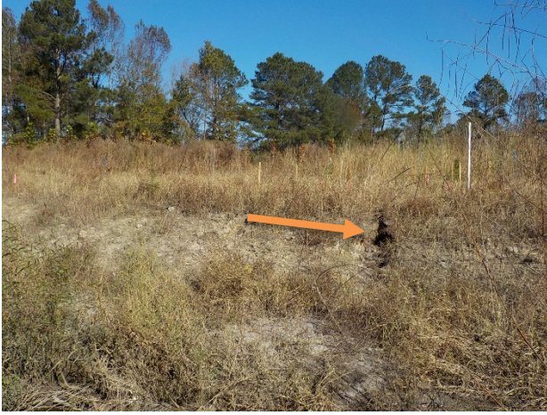
SPA1- Minor right bank erosion - Reach 5A @ Sta 17+40
