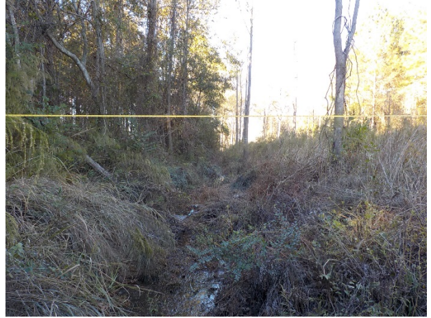
Reach 3C Looking Upstream Sta. 64+00- MY3 (11/7/2016)
