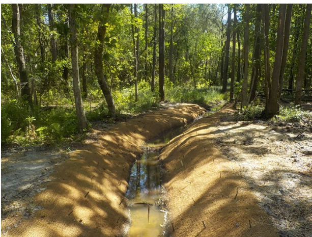
SPA2-MY2-2015 Repaired Structures (4/26/2016)
