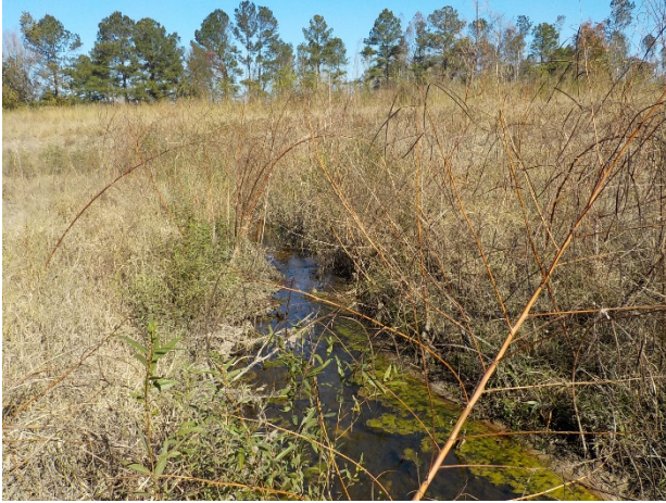
SPA5-MY2-2015 Reach 5A Repairs (11/8/2016)
