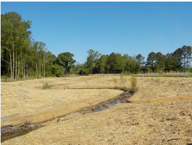
SPA5-MY2-2015 Reach 5A Repairs (4/26/2016)
