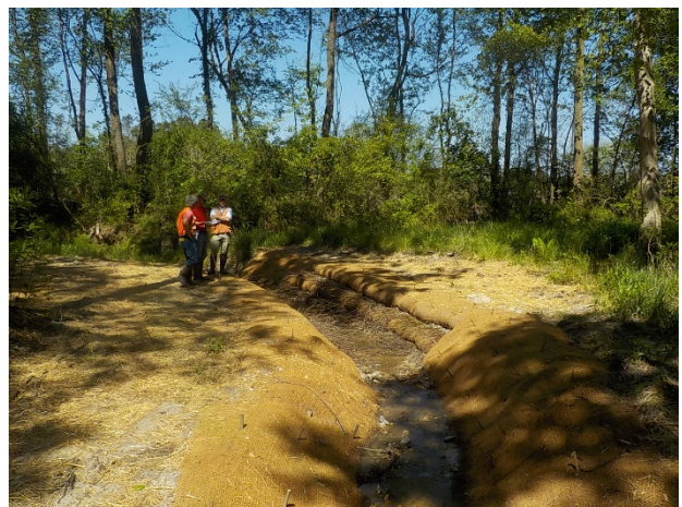
SPA2-MY2-2015 Repaired Structures (4/26/2016)
