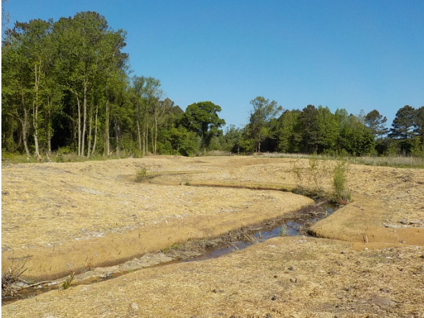
SPA5-MY2-2015 Reach 5A Repairs (4/26/2016)
