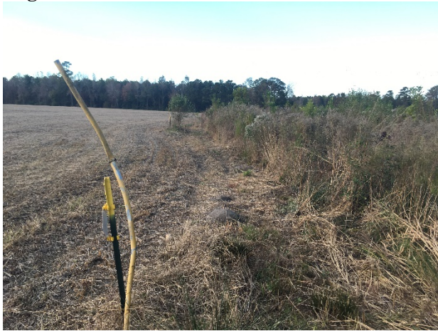
MY4 – VPA1 – Encroachment on Reach 1 & 3A at Sta. 1+00 to 9+97 (Reach 1) & 3+00 to 18+73 (Reach 3A)
