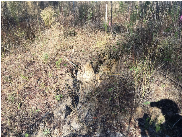
MY4 – VPA2 – Bare Area/ Head Cut Erosion Reach 5A at Sta. 17+40
