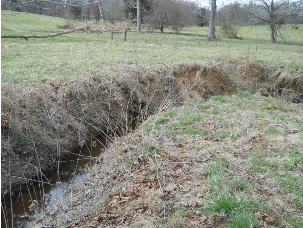
Photo 7. North Branch – Reach 1 (Restoration)
