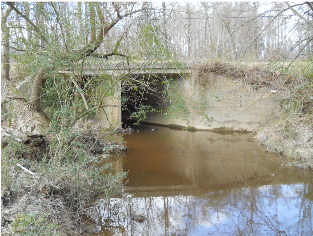
Photo 4. Double box culvert at downstream end of project
