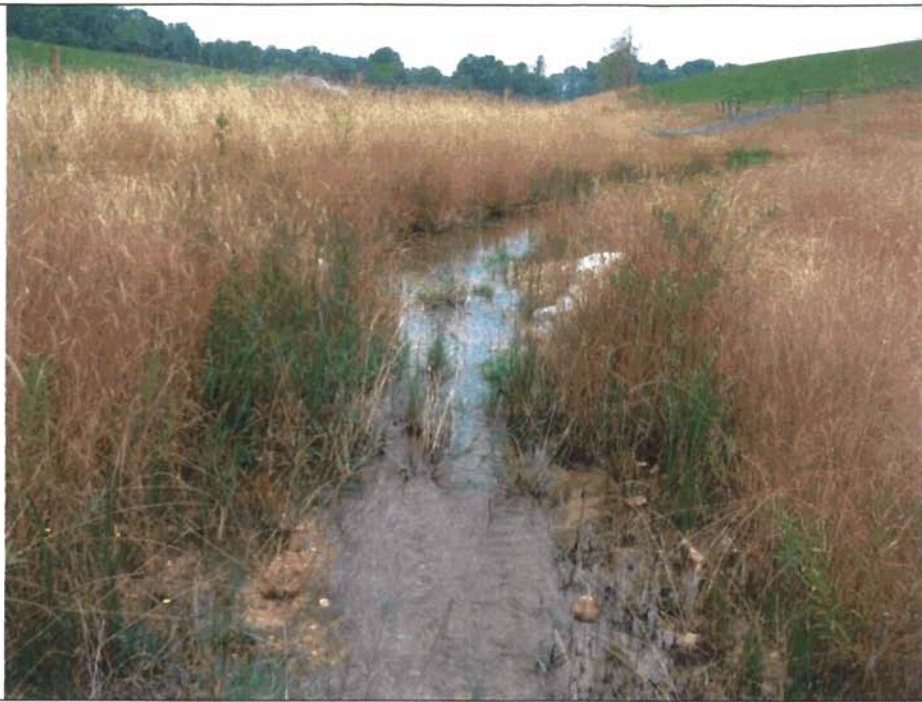
Photo 3: Looking downstream at channel
