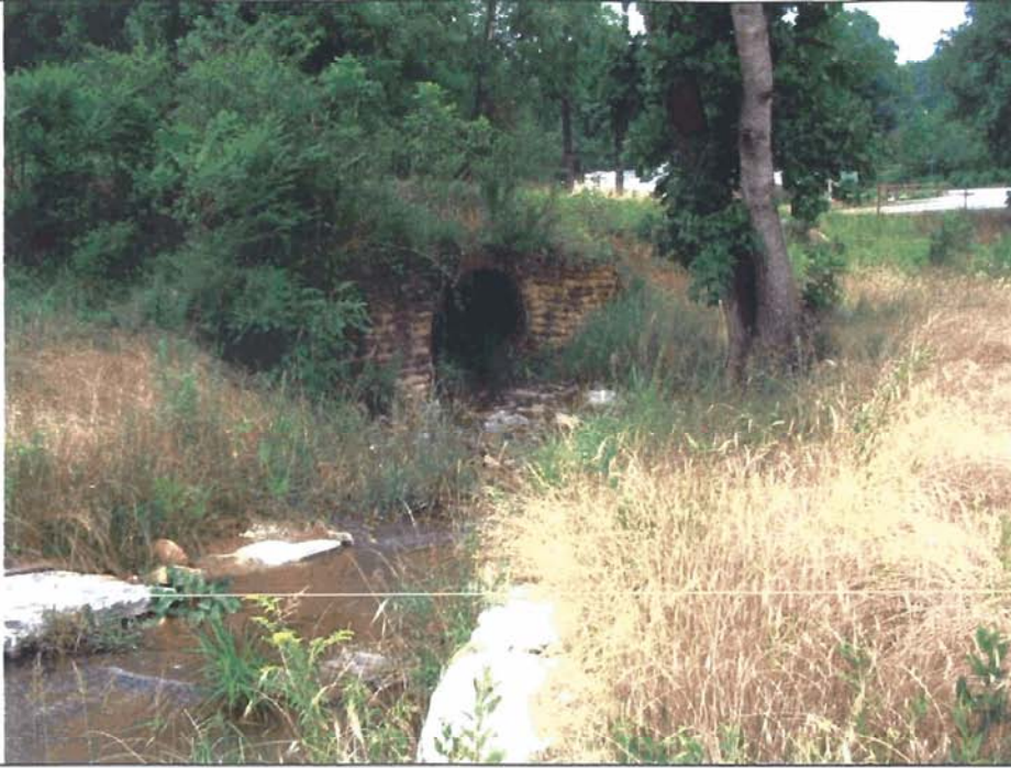
Photo 1: Looking upstream at culvert at top of project.
