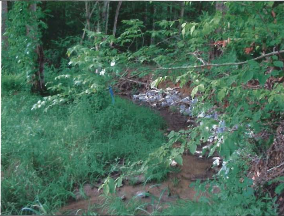
Photo 15: Looking downstream from right bank at rip-rap toe protection.
