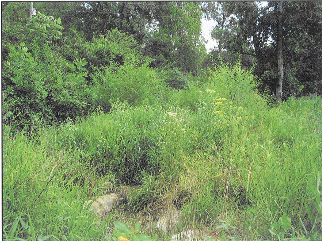
PHOTO 1: LOOKING UPSTREAM AT THE CULVERT AT TOP OF PROJECT.
