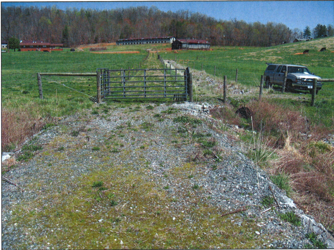
PHOTO 5: LOOKING AT LEFT BANK AT DRAINAGE SWALE ENTERING CHANNEL FROM LEFT SIDE.
