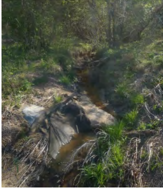
Photo Point 25 – UT-2 to Walton Crawley Branch
