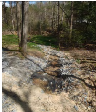
Photo Point 30 – UT-2 to Walton Crawley Branch
