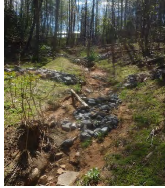
Photo Point 32 – UT-2 to Walton Crawley Branch
