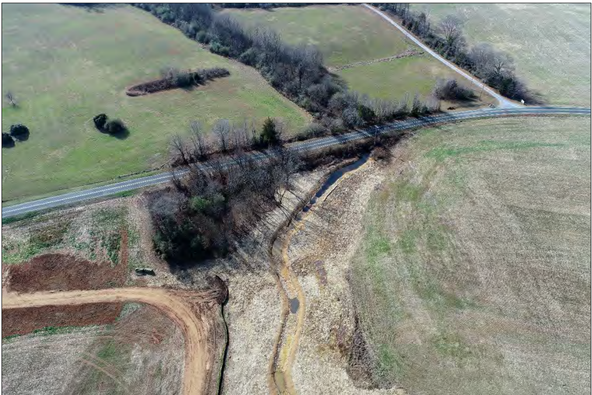
Glen Branch / Site outfall - 01/15/2022
