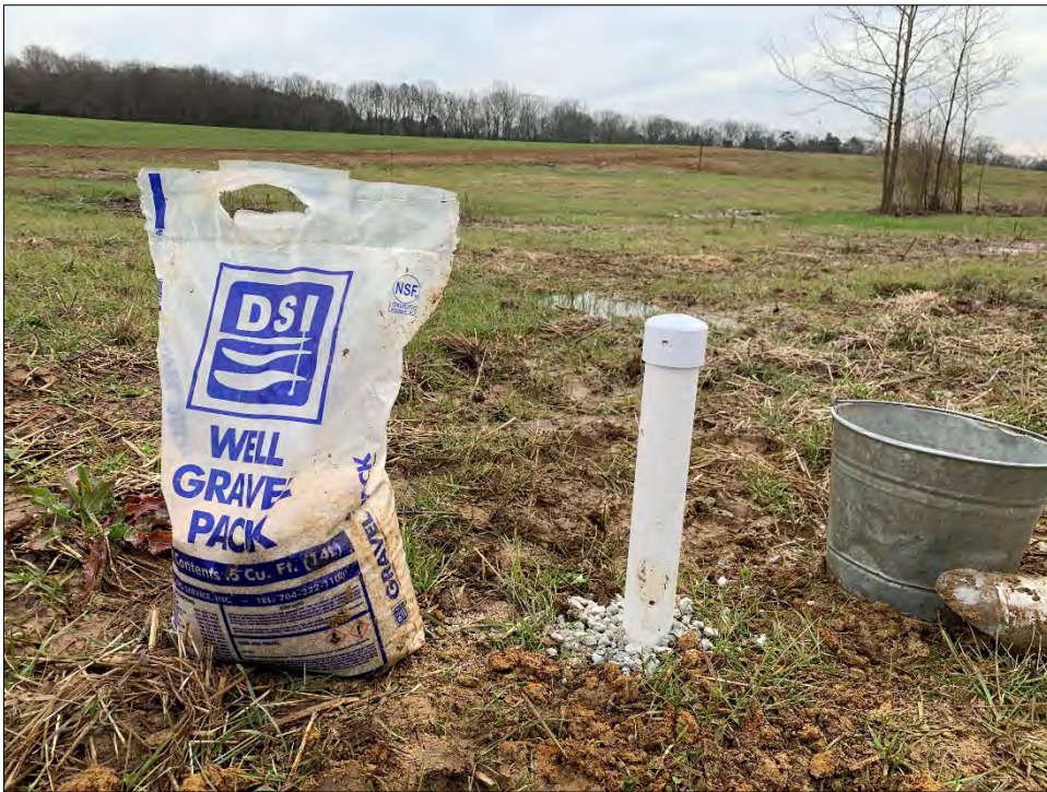
Ground Water Gauge Install - 02/02/2022
