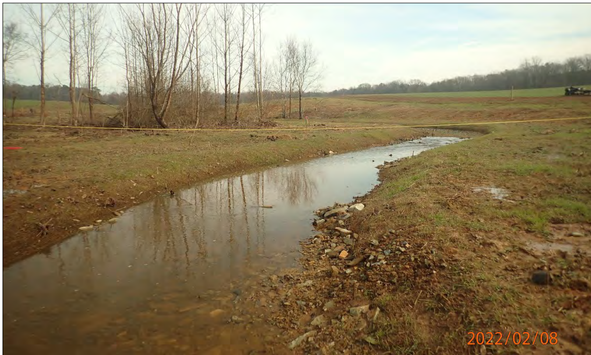
Cross sections 5, Glen Branch - 02/08/2022
