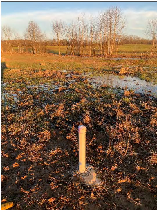
Ground Water Gauge Install - 02/02/2022
