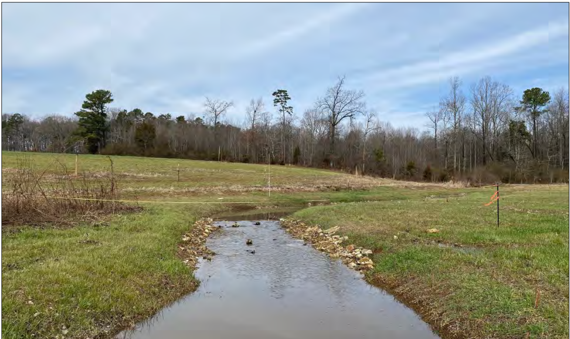
Cross sections 11, Glen Branch - 02/08/2022
