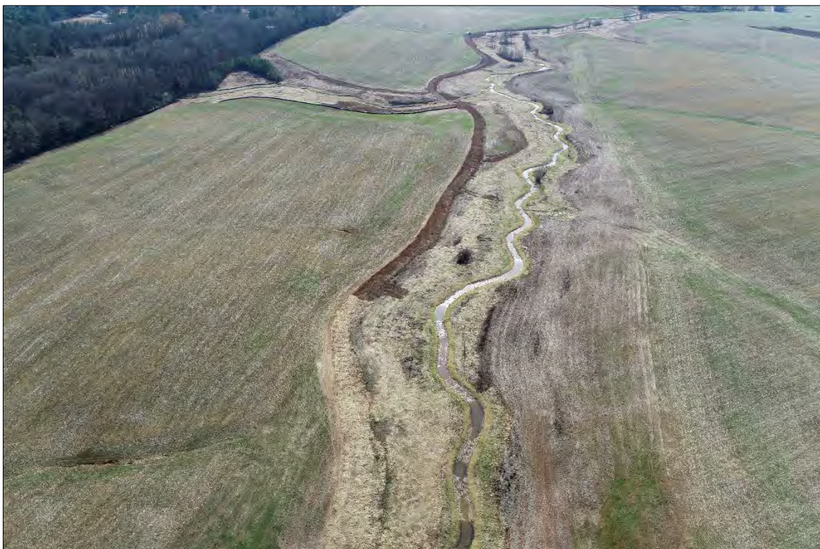
Glen Branch, upper extent, looking south - 01/15/2022
