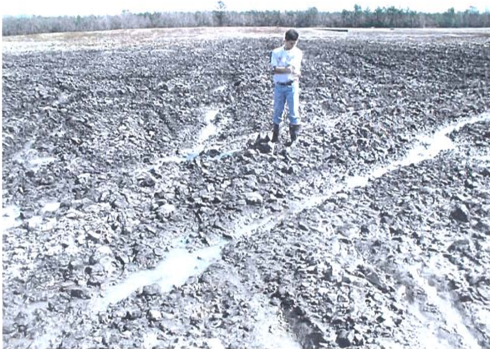
Photo 4. Restoration area after grading and tillage operations were completed.
