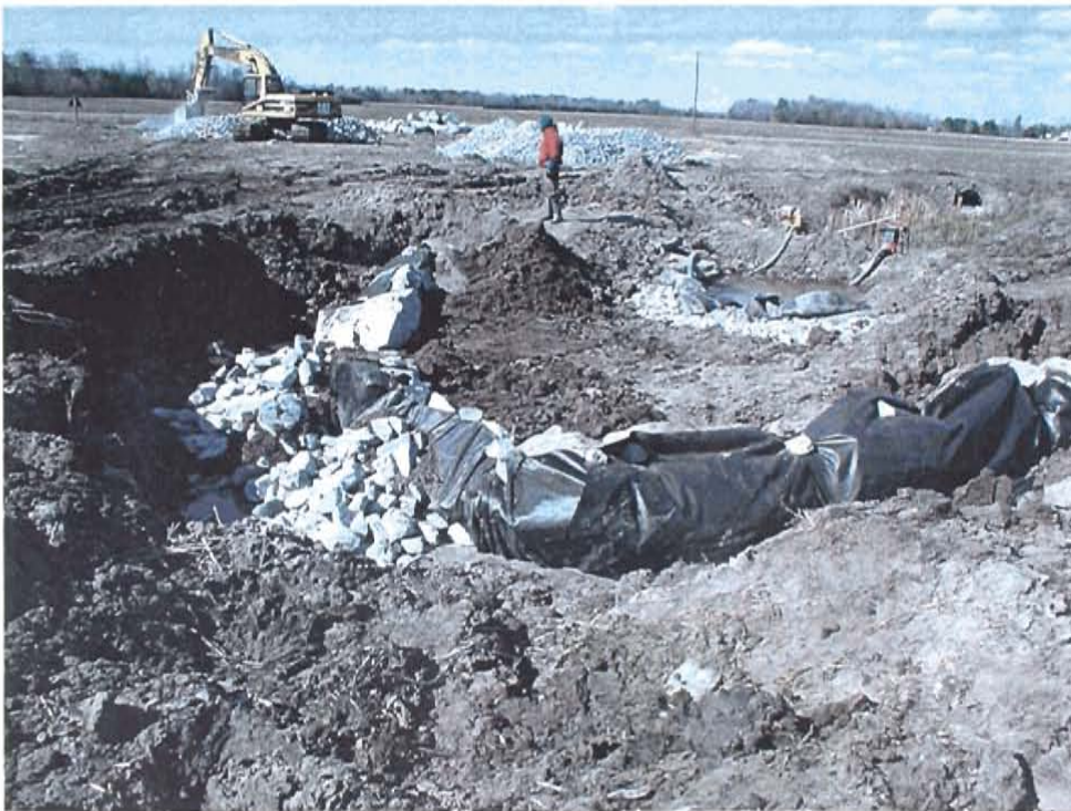
Photo 8. Sealing of cross-vane structure.
