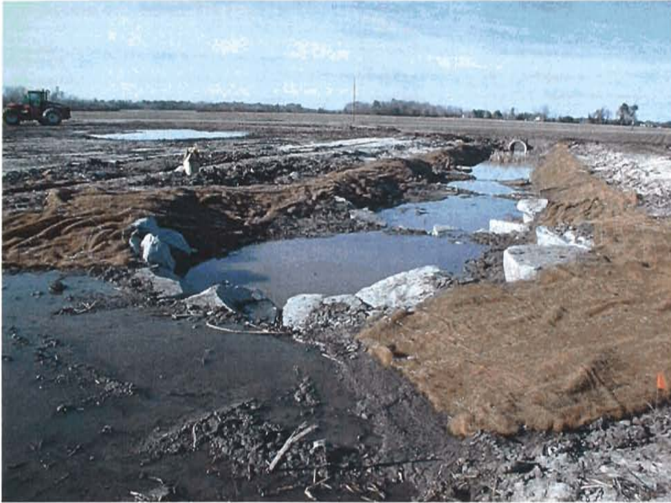
Photo 9. Completed cross-vanes with protective erosion control matting.
