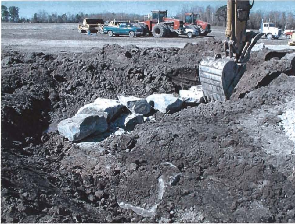
Photo 7. Cross-vane construction with footer rocks.
