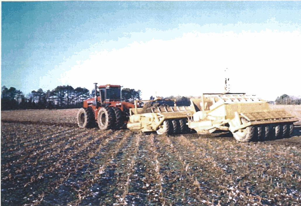
Photo 1. Site grading with laser level equipped pan excavator.
