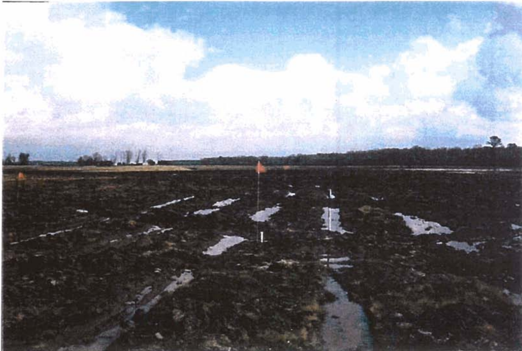
Photo 17. Monitoring plot #3 on March 20,2002 after rainfall event.
