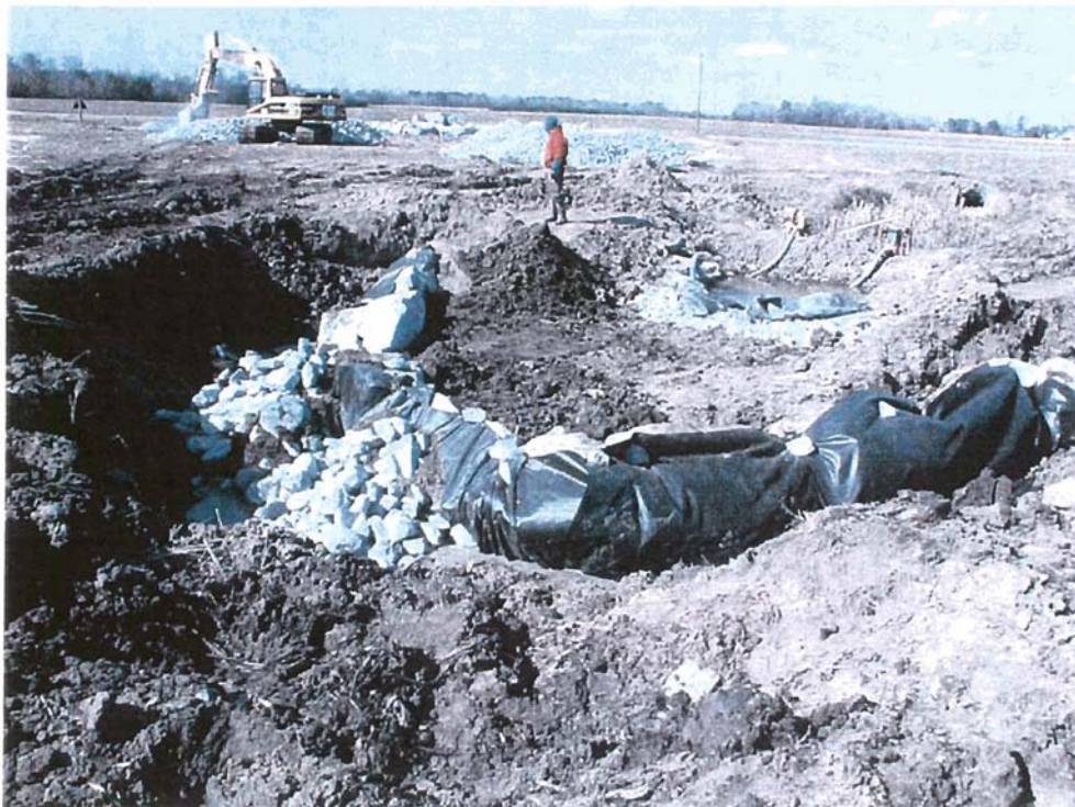
Photo 8. Sealing of cross-vane structure.
