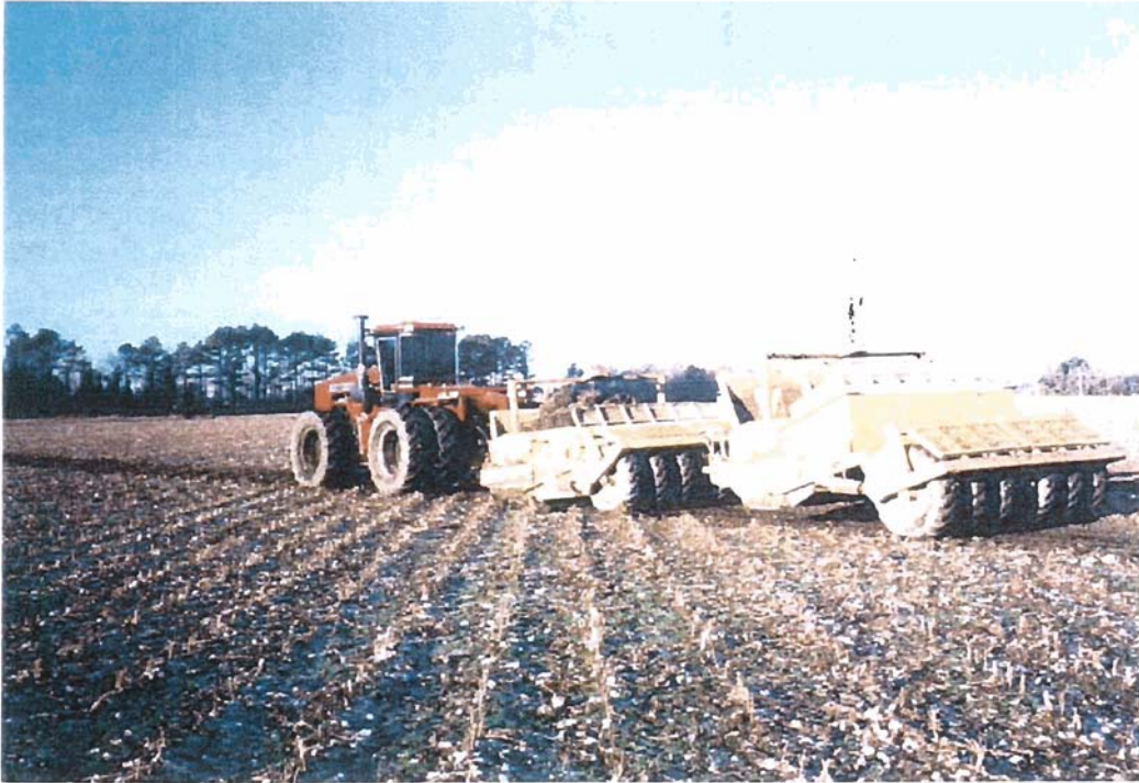
Photo 1. Site grading with laser level equipped pan excavator.
