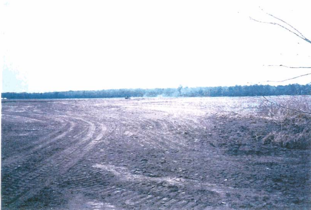
Photo 2. Completed grading on the west side of the site.
