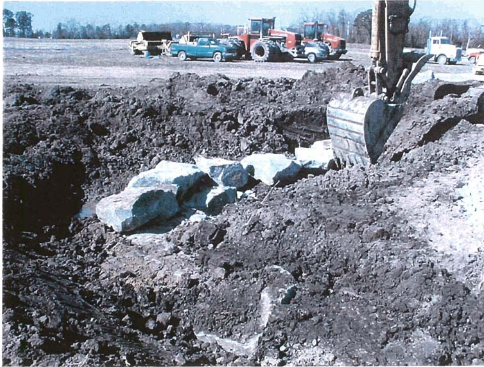
Photo 7. Cross-vane construction with footer rocks.
