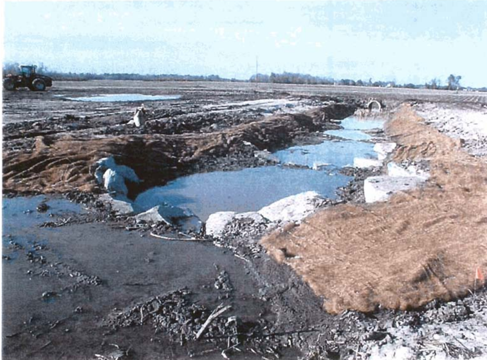
Photo 9. Completed cross-vanes with protective erosion control matting.
