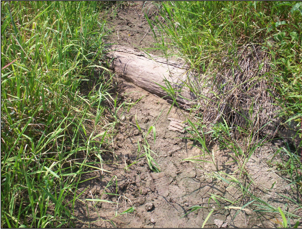
Photo 7 Station 59+50 Reach 1 upstream. Log vane.
