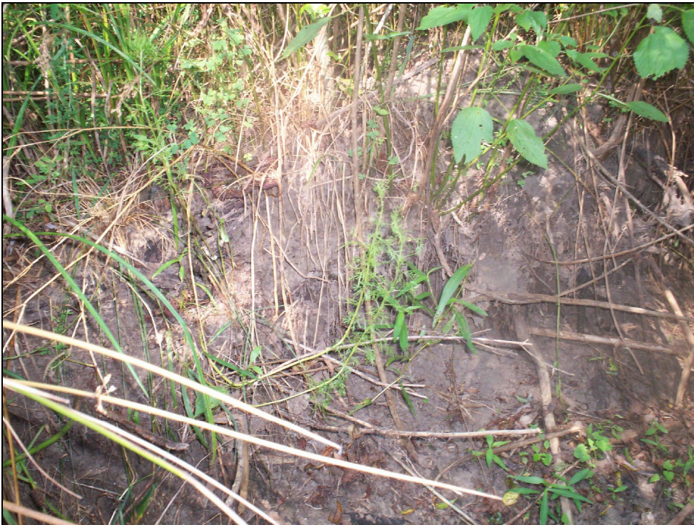
Photo 8 Station 39+74 Reach 1 left bank. Root wad.
