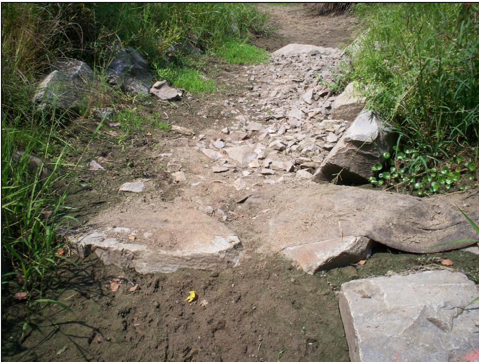
Photo 4 Station 71+60 Reach 1 upstream. Constructed Riffle.
