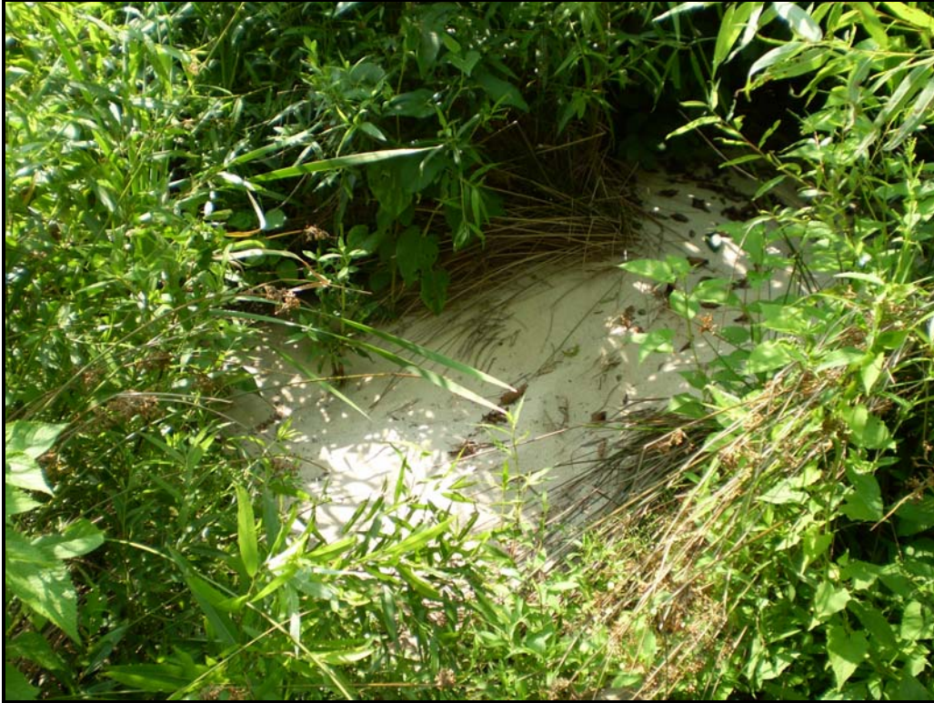
Sediment/sand entering channel @ station 32+90 (Reach 1) causing potential aggradation in channel.
