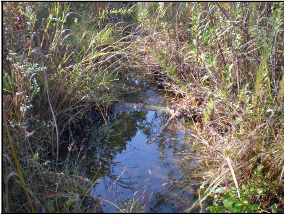
Tapp – Log weir facing upstream (typ.)
