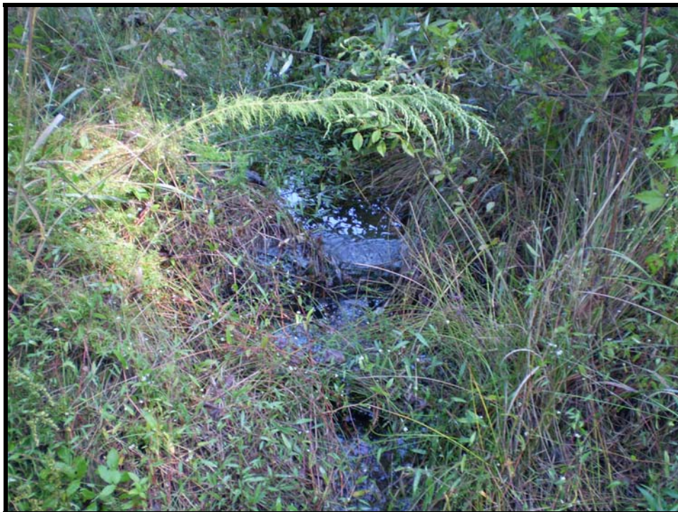
Tapp – Log weir facing upstream (typ.)
