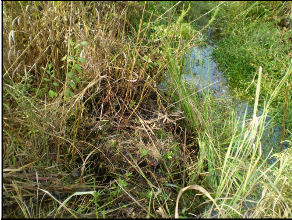
Reach 1, Station 16+75 - Erosion behind rootwad (PA1)
