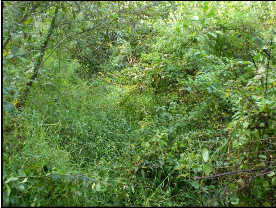
Reach 2 – Heavy vegetation in channel throughout reach, restricting flow (PA3)
