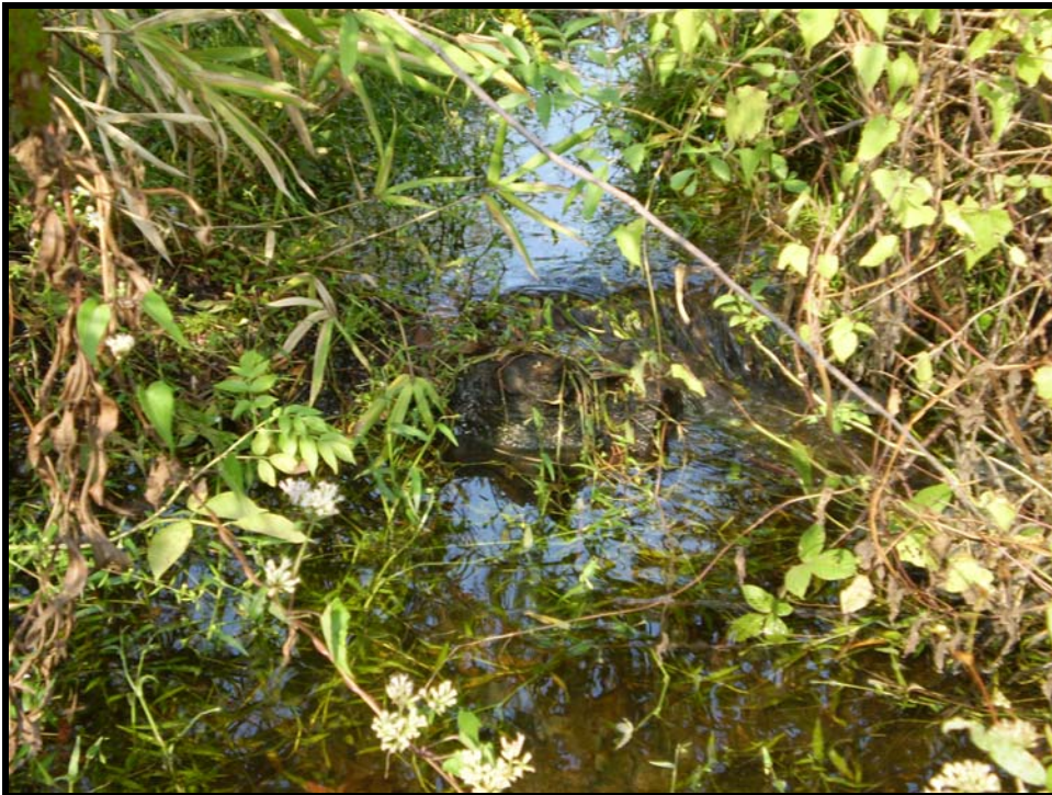
Cole - Log weir facing upstream (typ.)
