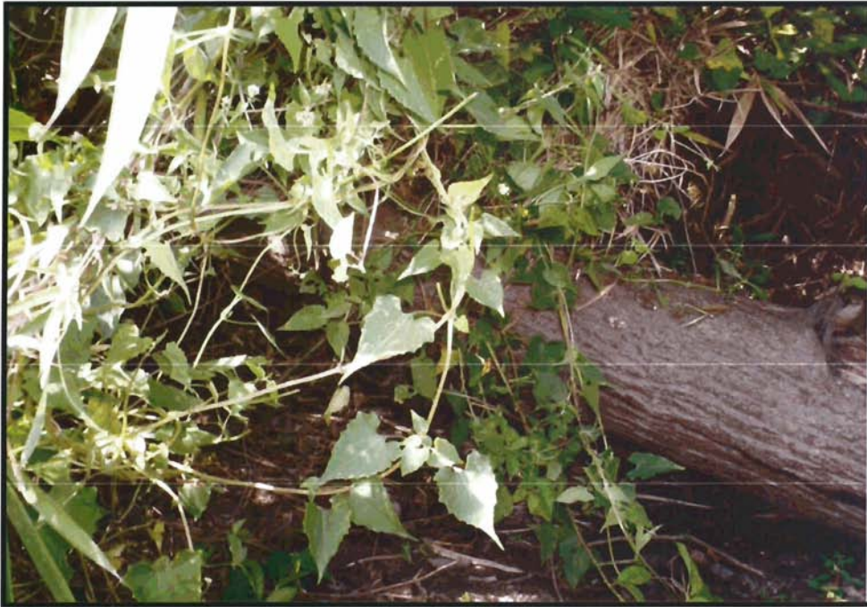
SPA 2. Undercutting at log vane STA 43+80.
