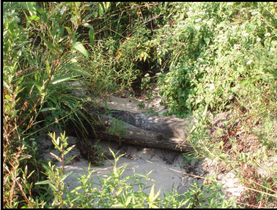
Log weir @ station 3+40 facing upstream
