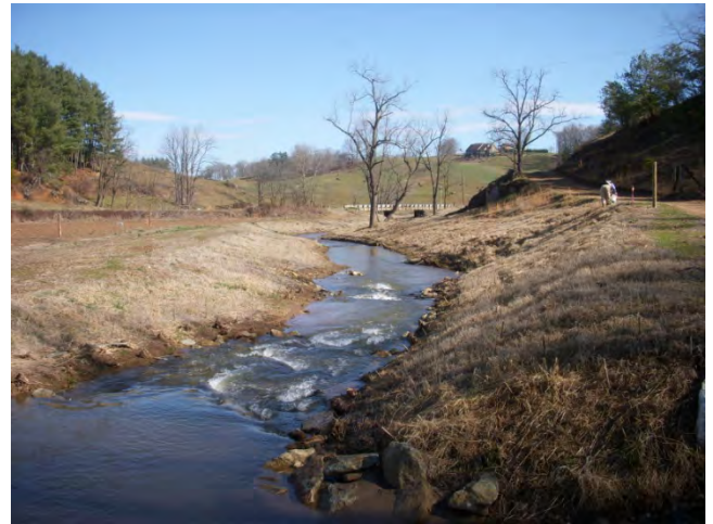
PS46, Mainstem facing downstream
