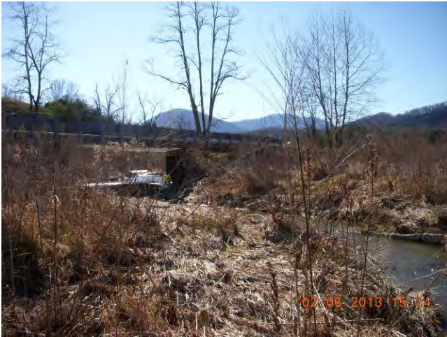
PS49, Mainstem facing downstream
