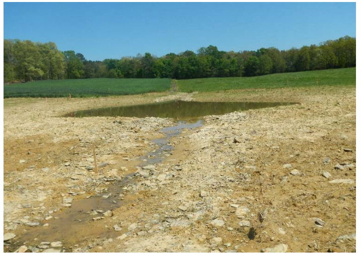
Photo Point 51 – looking upstream at pond (04/23/2014)
