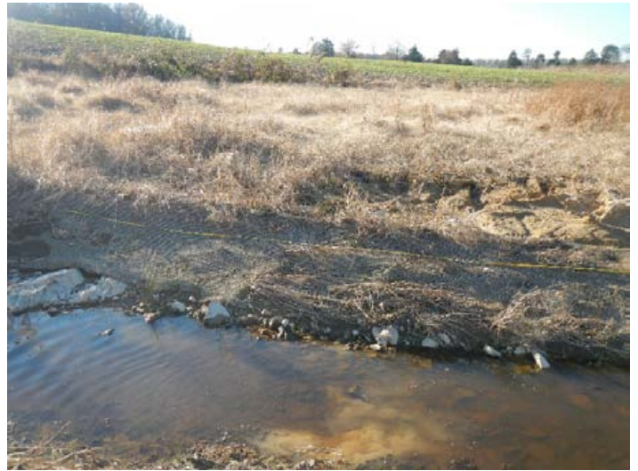
AOC-2: Bare bank on Norkett Branch Reach 1 left bank, 12-1-2014
