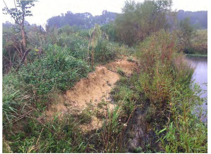
Bare Bank: Norkett Branch Station 132+75) – 10/17/2018
