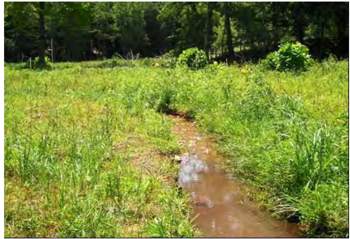
Sta. 117+94 Looking Downstream
