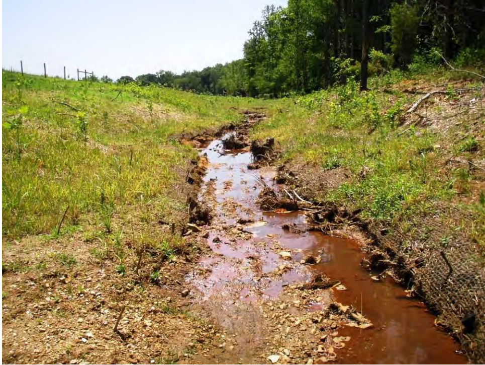
Photo B15 – Photo Station S15 Reach 2 cross-section 3 looking downstream (6/27/2012)
