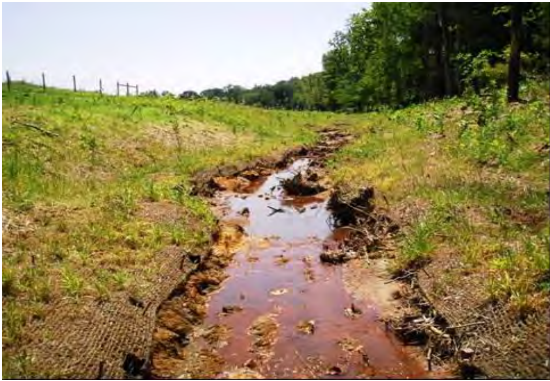
Sta. 107+60 Looking Downstream
