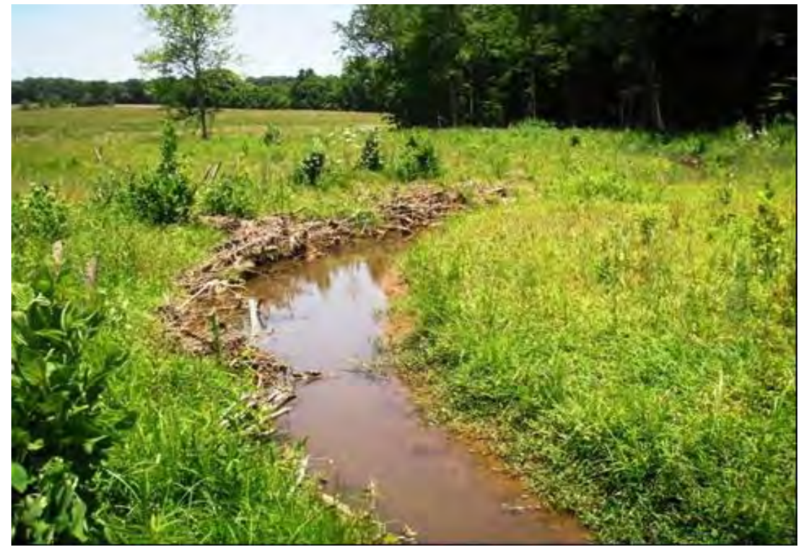
Sta. 314+59 Looking Downstream
