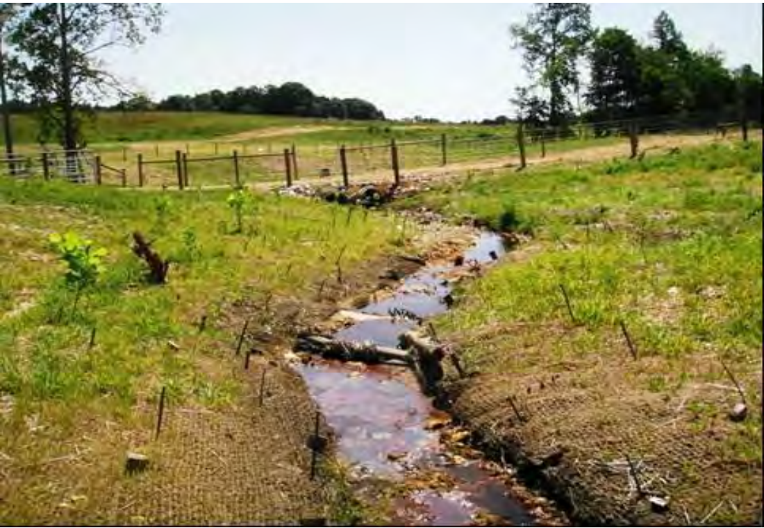
Sta. 204+01 Looking Downstream
