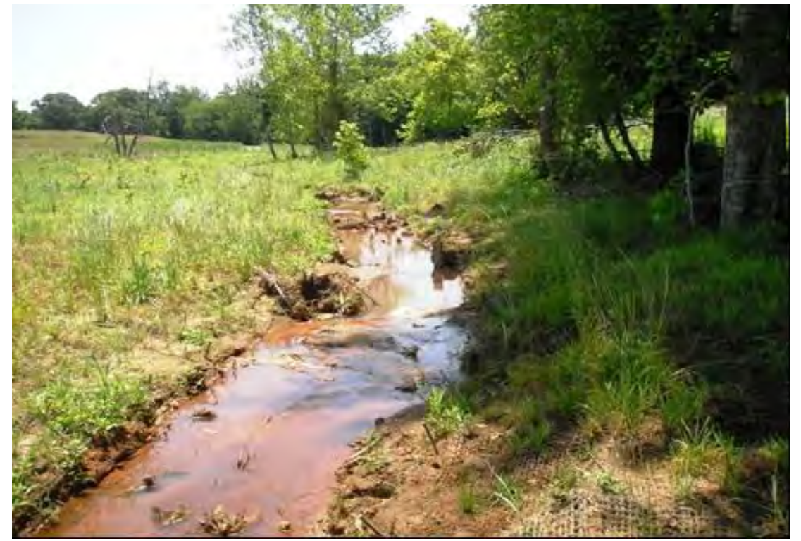
Sta. 114+55 Looking Downstream
