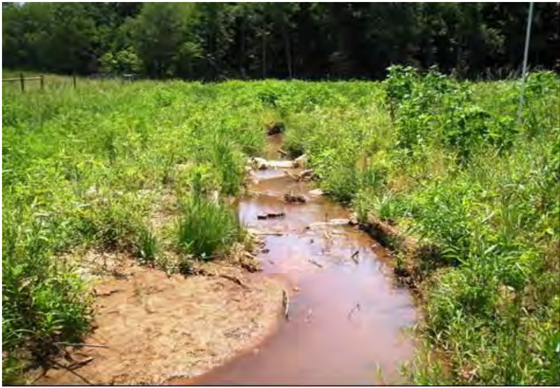
Sta. 120+73 Looking Downstream
