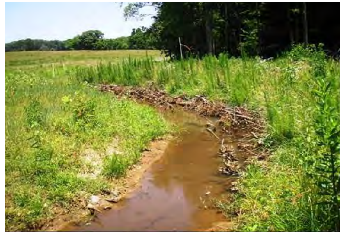
Sta. 317+28 Looking Downstream
