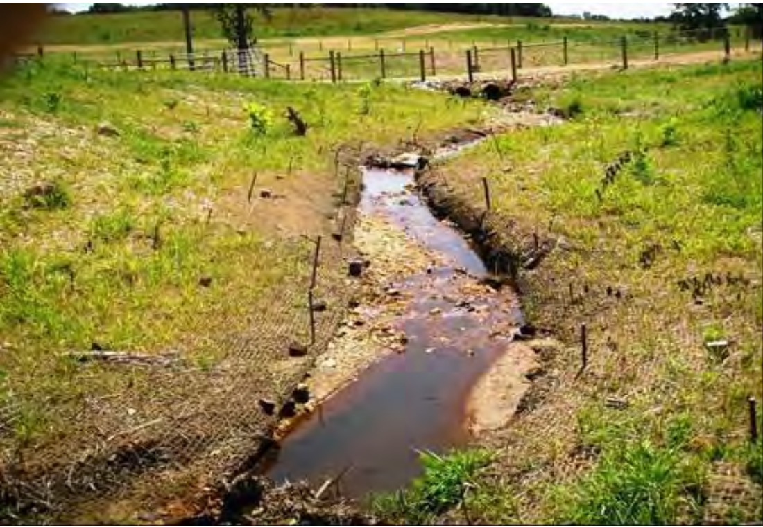
Sta. 203+75 Looking Downstream
