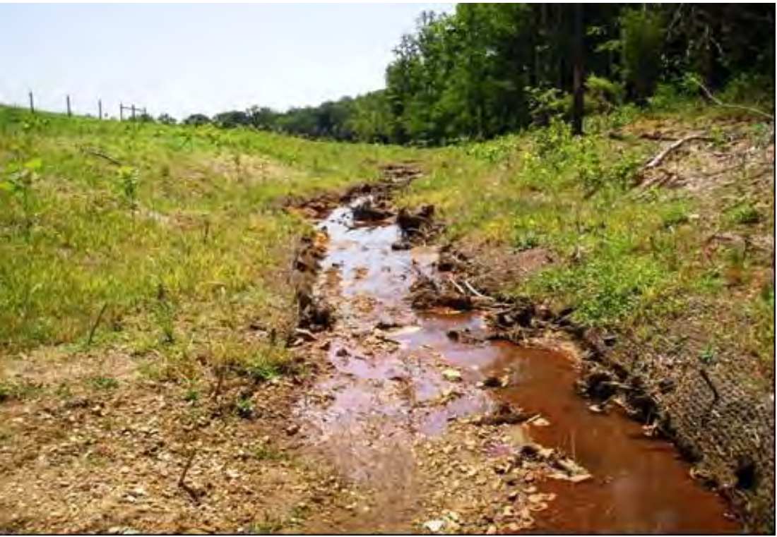
Sta. 107+28 Looking Downstream
