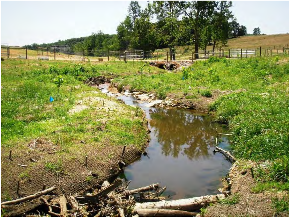
Photo B14 – Photo Station S14 Reach 1 cross-section 2 looking downstream (6/27/2012)
