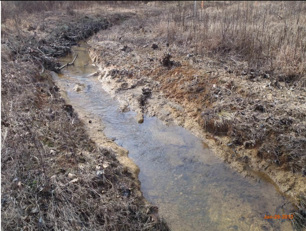
1-S Reach 1 Sta. 305+50 – Riffle Degradation
